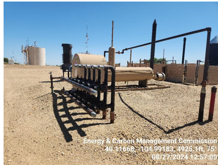
Photo 12 Flow line manifold & Horizontal Heated Separator.
