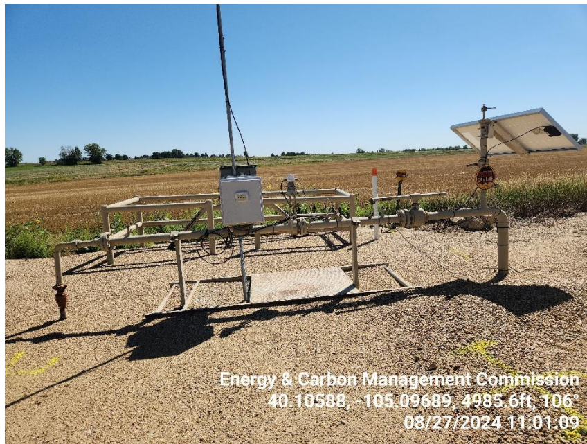
Photo 5 Gas Meter Run
