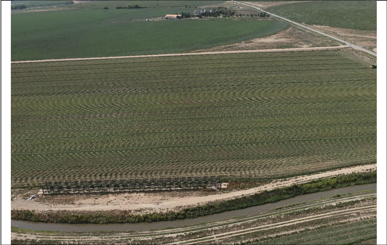
In View – Well, Access Road, Flowline
