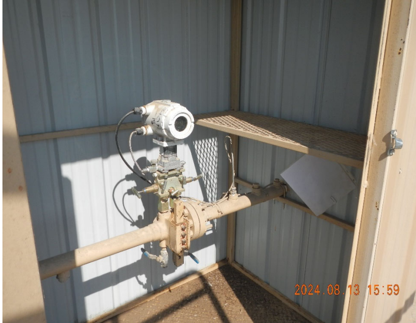
3. Digital gas meter inside meter shed.
