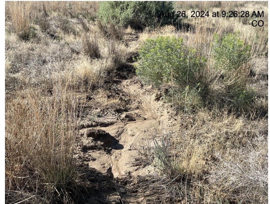
Photo # 6266 Erosion & transport of sediment off location & into vegetated areas/failure to minimize erosion & the transport of sediment off location
