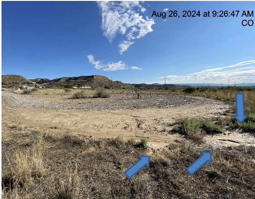
Photo # 6259 Erosion & transport of sediment off location & into vegetated areas/failure to minimize erosion & the transport of sediment off location (S/SW edge of pad near wellhead)
