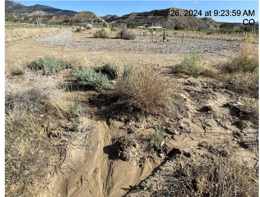
Photo # 6264 Erosion & transport of sediment off location & into vegetated areas/failure to minimize erosion & the transport of sediment off location (S/SW edge of pad near wellhead)
