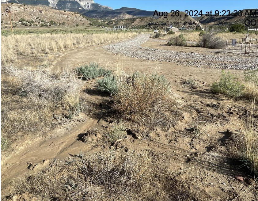
Photo # 6263 Erosion & transport of sediment off location & into vegetated areas/failure to minimize erosion & the transport of sediment off location (S/SW edge of pad near wellhead)
