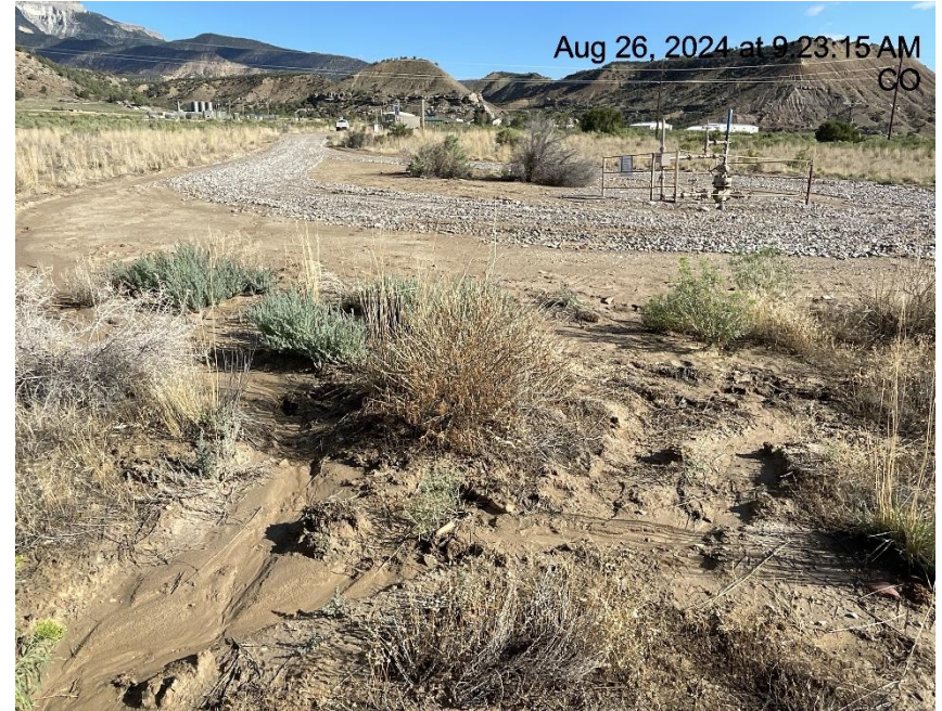
Photo # 6262 Erosion & transport of sediment off location & into vegetated areas/failure to minimize erosion & the transport of sediment off location (S/SW edge of pad near wellhead)
