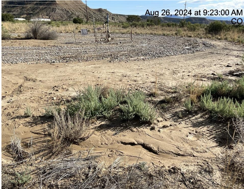
Photo # 6261 Erosion & transport of sediment off location & into vegetated areas/failure to minimize erosion & the transport of sediment off location (S/SW edge of pad near wellhead)
