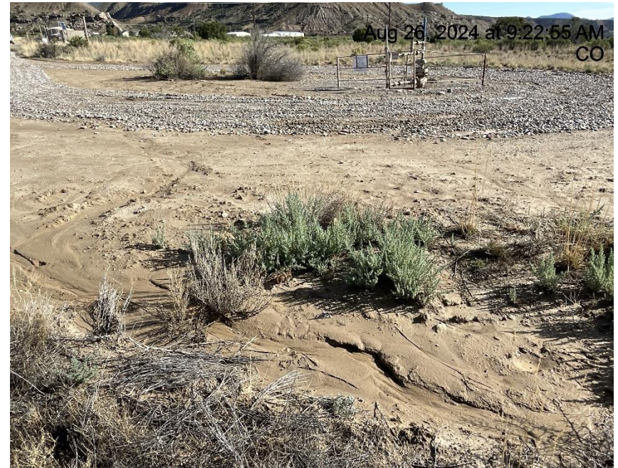
Photo # 6260 Erosion & transport of sediment off location & into vegetated areas/failure to minimize erosion & the transport of sediment off location (S/SW edge of pad near wellhead)
