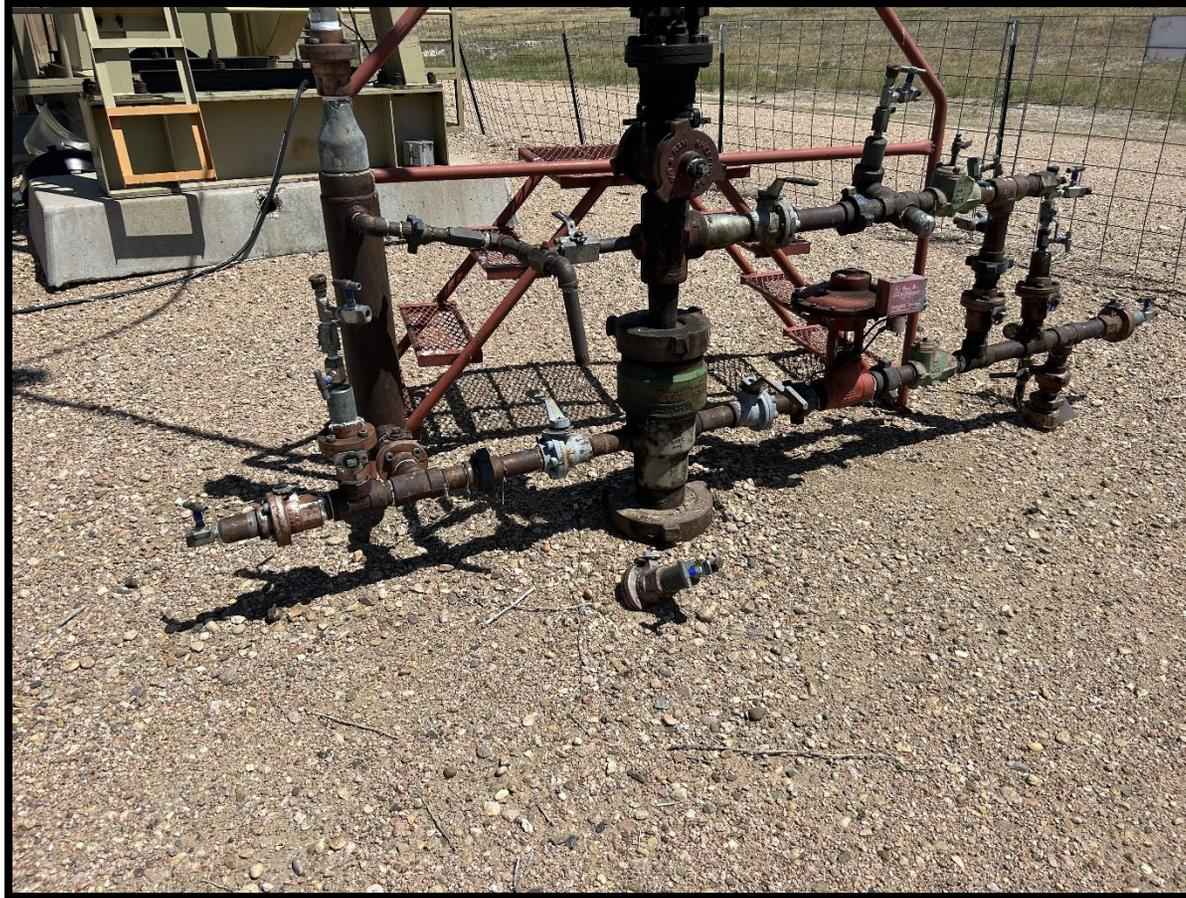
**CA:** Stained Soil at Wellhead: For localized stained soils or oily waste - ""Properly dispose of oily waste in accordance with 907.e."" Securely fasten all valves, pipes, and fittings to ensure good mechanical condition, inspect at regular intervals and maintain in good mechanical condition per Rule 605.d.
