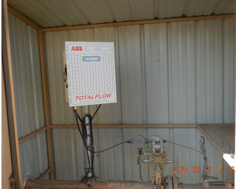
5. Digital gas meter inside remote meter shed.
