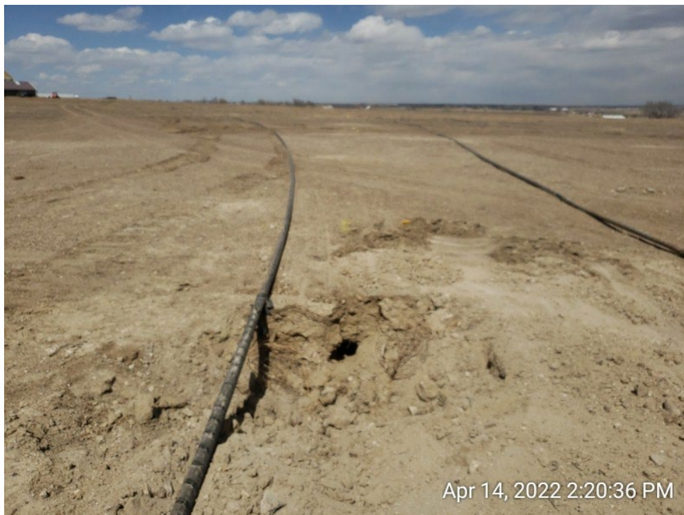
#1A – Howard A27-7 – Flowline Cut and Cap at Wellhead – 7FL01@2.0' – Facing NE – Flowline in good condition with no damage or corrosion – Sample Submitted for Lab Analysis – PID 0.4ppm
