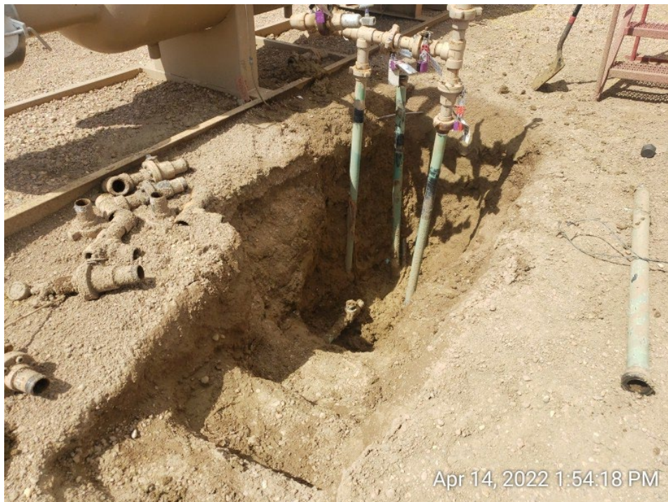
#1F – Howard A27-7 – Flowline Cut and Cap at Separator Tie-in – 7FL06@5.0' – Facing NW – No Impacts Noted – Sample Submitted for Lab Analysis – PID 0.7ppm
