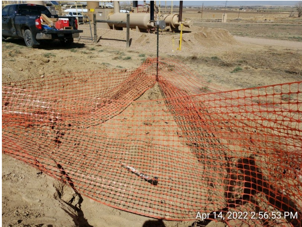
#1E – Howard A27-7 – Flowline Cut and Cap – 45' Abandoned-in-Place Leading to Separator Tie-in - 7FL05@3.0' – Facing NE – No Impacts Noted – Sample Submitted for Lab Analysis – PID 0.2ppm
