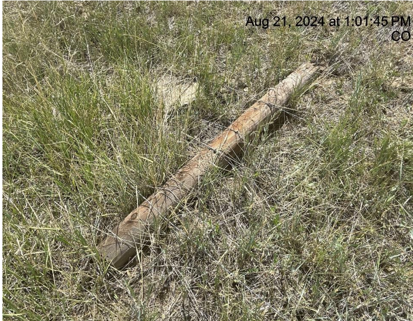
Photo # 5861 Barbed wire fence needs maintenance/wildlife hazard
