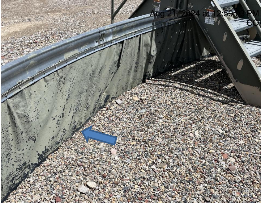
Photo # 5857 Hole in liner/liner needs maintenance
