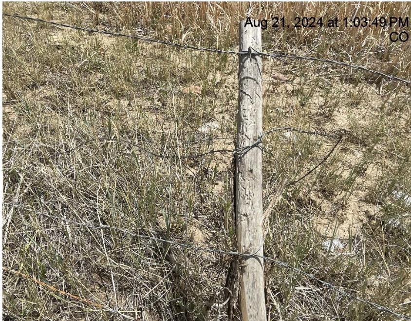
Photo # 5867 Barbed wire fence needs maintenance/wildlife hazard
