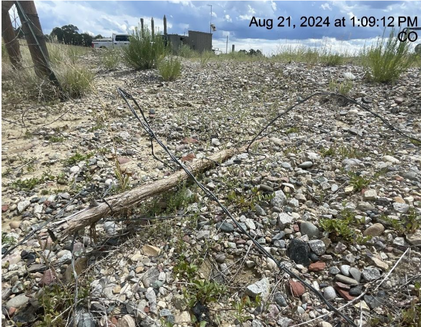
Photo # 5871 Barbed wire fence needs maintenance/wildlife hazard
