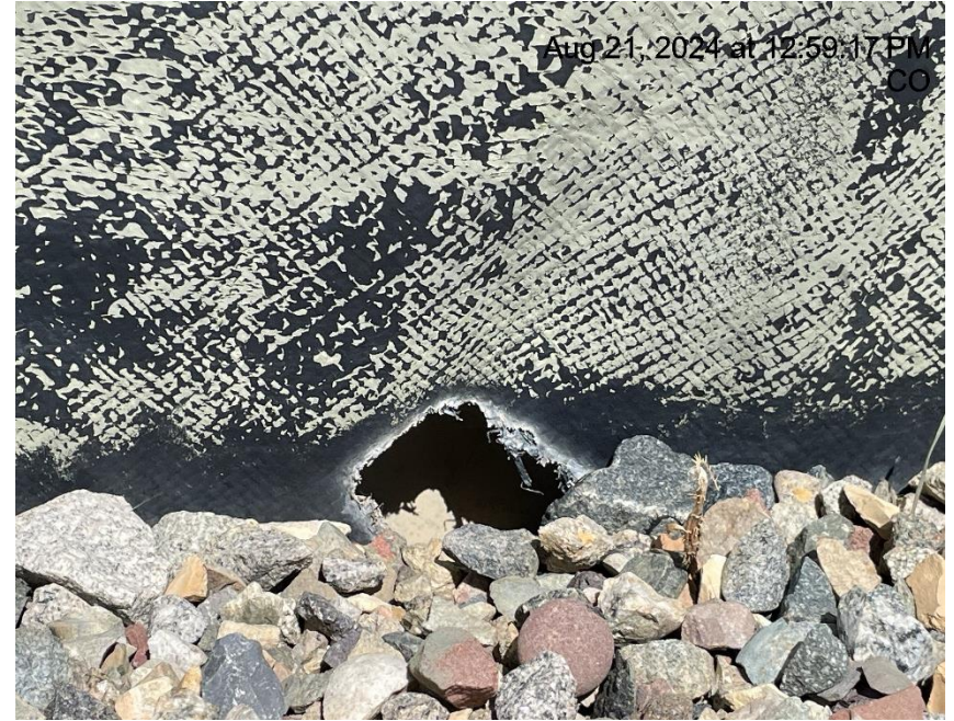
Photo # 5858 Hole in liner/liner needs maintenance
