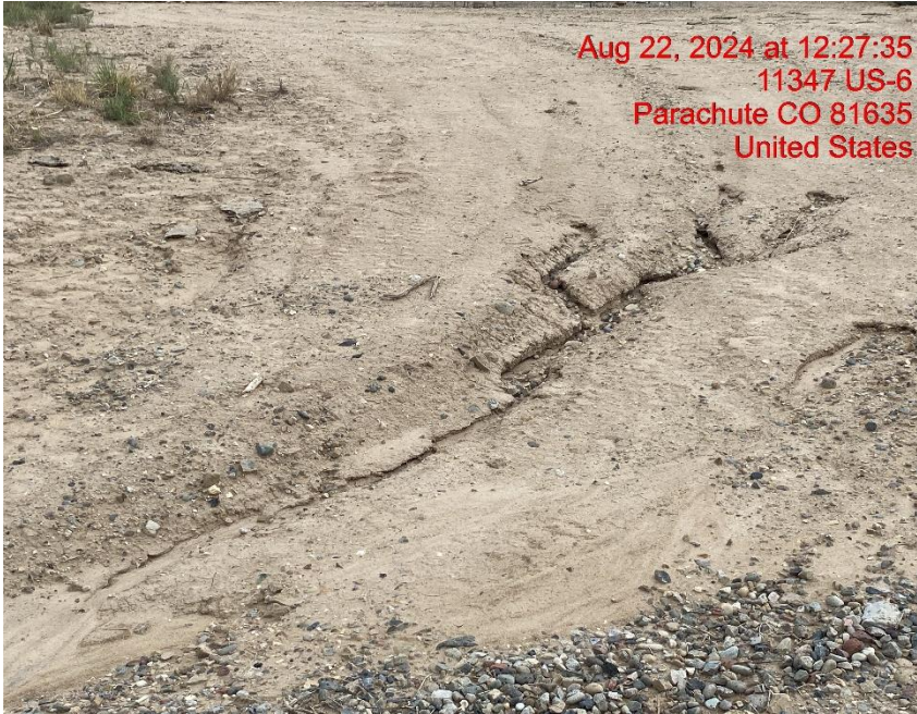
Insufficient Erosion Control – Photo #02995
