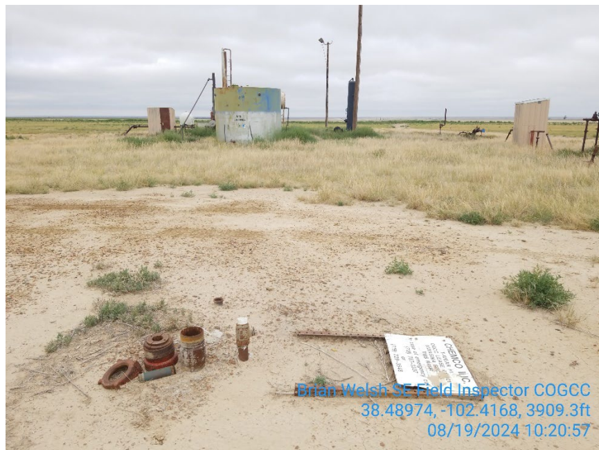
Well is plugged but not cut and capped
