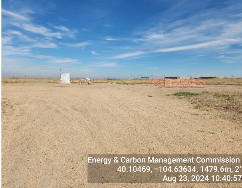
Photo 1: Location from entrance, gas meter
