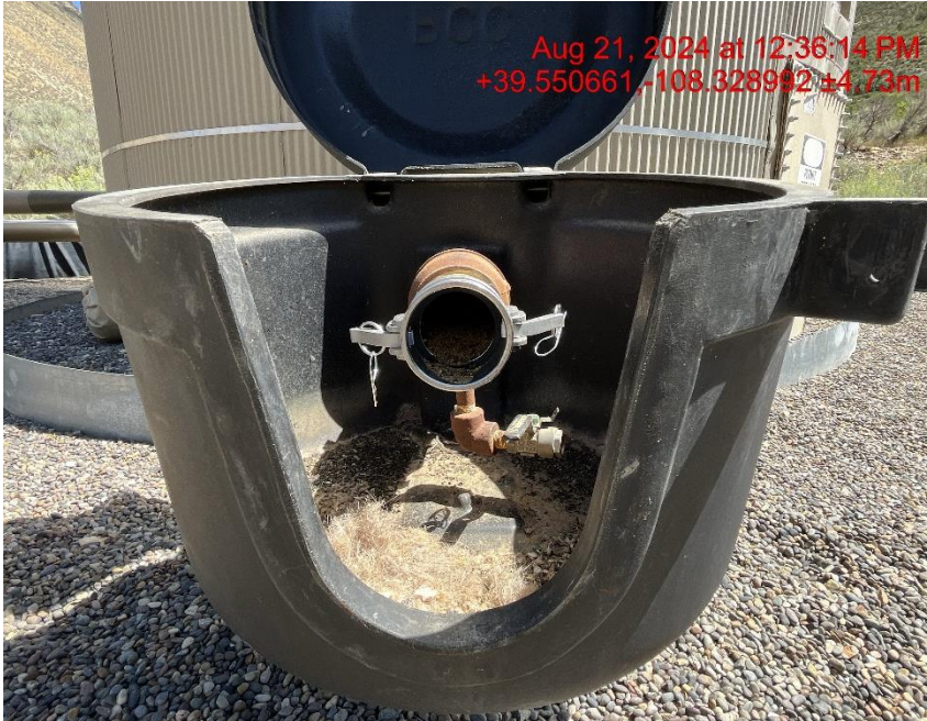
Open ended load line - Photo #04859
