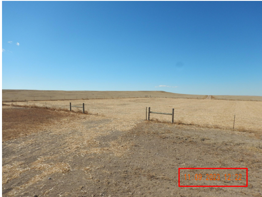
Photo 1. Photo taken from the eastern entrance of location on 11/9/2023, facing Southwest. Photo illustrates the Operator has performed final reclamation activities to reseed the location with the evidence of straw crimped mulch.
