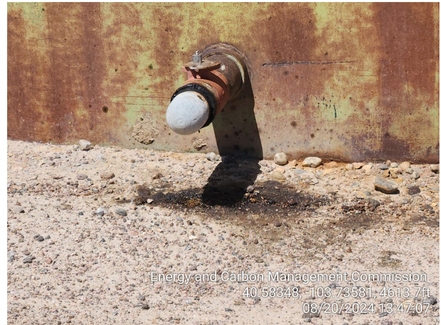
Photo 6 – Stained Soil at Southeast Tank Loadline Valve
