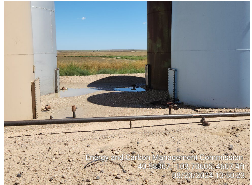
Photo 18 – Unmarked Risers at Tanks
