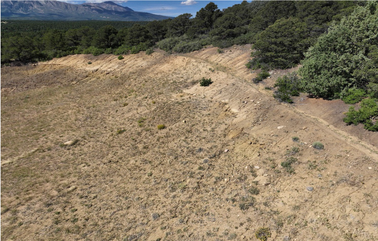
Photo 5. Drone aerial photo facing southwest toward the cut slope. There are some signs of erosion in this area.
