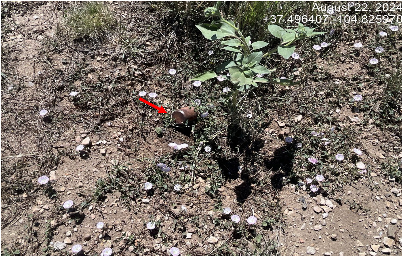
Photo 7. There is field bindweed throughout the location that will need to be controlled. There is a capped flowline riser that needs to be removed or cut 3' below the surface.
