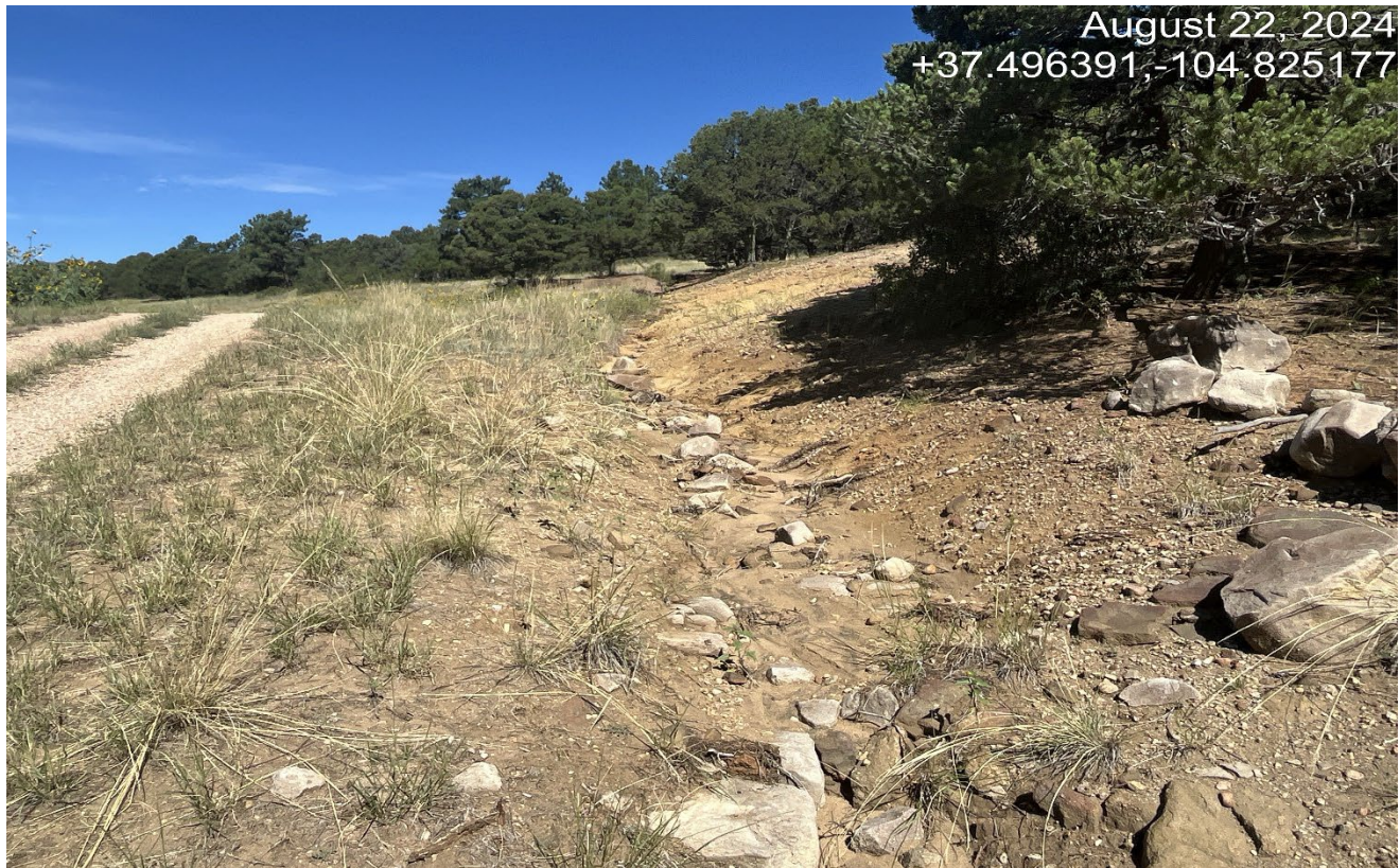
Photo 2. Facing northwest. The cut slope is not stabilized and has signs of erosion.
