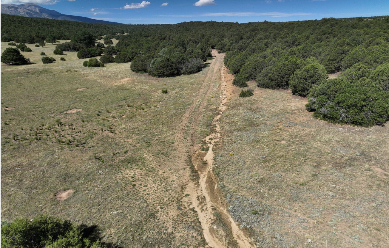
Photo 1. Drone aerial photo facing west toward the access road. There is sediment being deposited on the road from the ditch along the road side further up the road.
