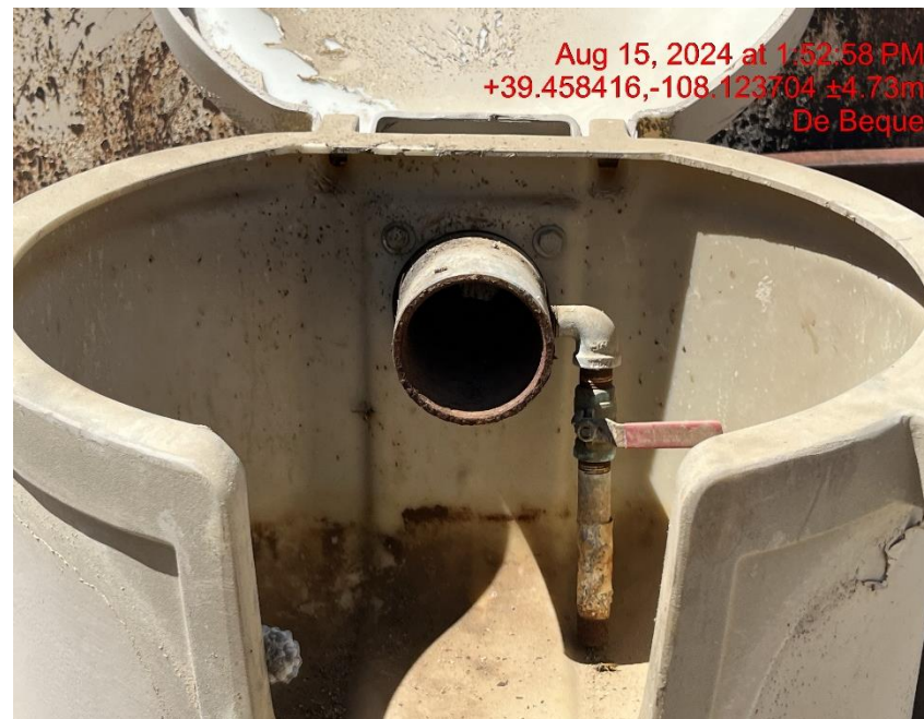
Open ended load line - Photo #04640
