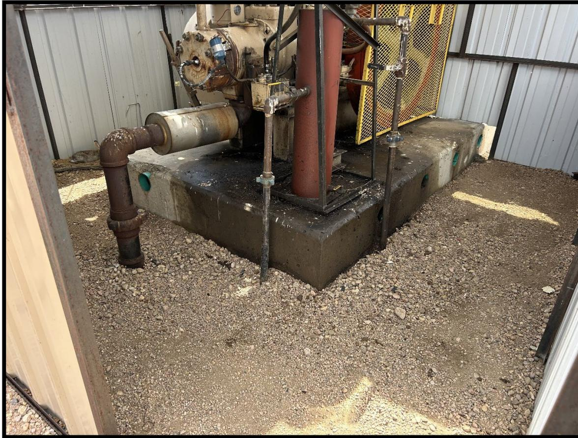
**CA:** Stained Soil at Engine and Exhaust, For localized stained soils or oily waste - Properly dispose of oily waste in accordance with 907.e
