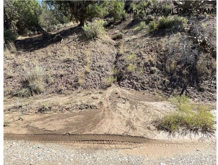
Photo # 5603 Erosion & transport of sediment/insufficient BMP's along spur road to location/sediment migration from slope onto spur road in multiple areas
