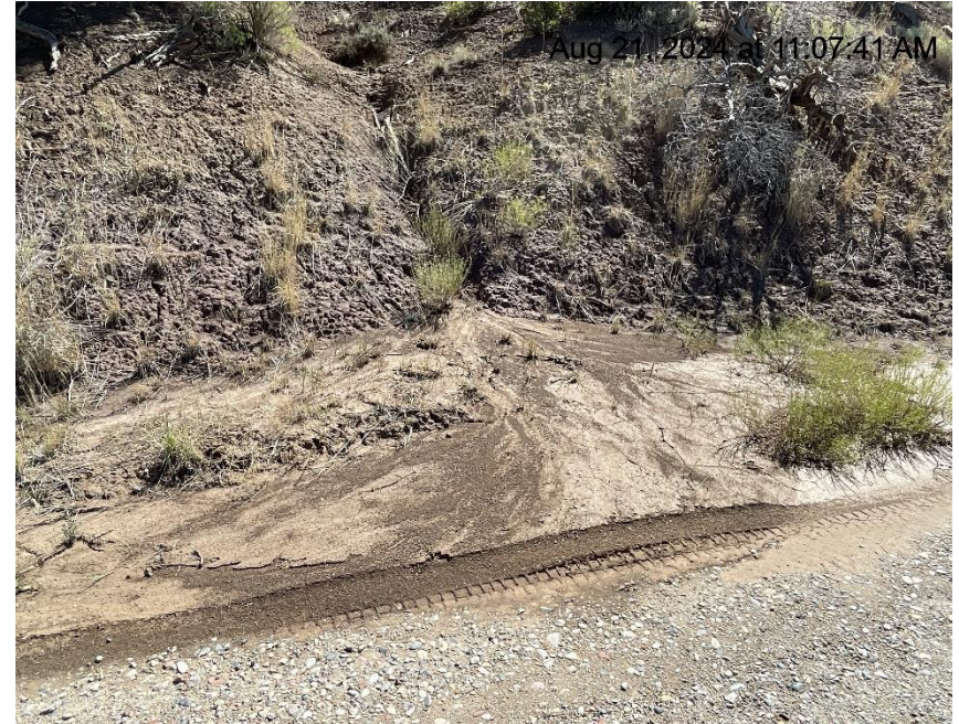
Photo # 5605 Erosion & transport of sediment/insufficient BMP's along spur road to location/sediment migration from slope onto spur road in multiple areas
