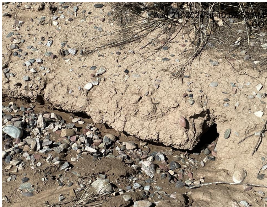
Photo # 5600 Tunnel erosion & transport of sediment off location
