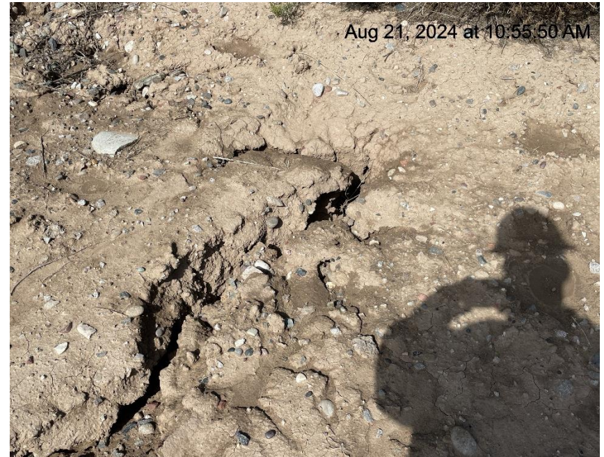
Photo # 5593 Tunnel erosion & transport of sediment off location
