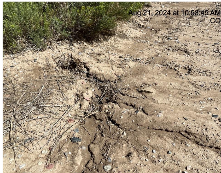
Photo # 5597 Tunnel erosion & transport of sediment off location
