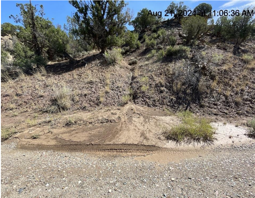
Photo # 5604 Erosion & transport of sediment/insufficient BMP's along spur road to location/sediment migration from slope onto spur road in multiple areas
