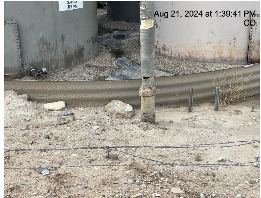
Photo # 5964 Barbed wire fence needs maintenance/wildlife hazard
