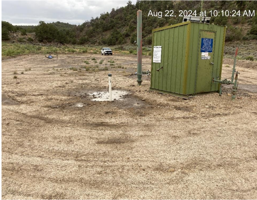
Location from Northwest corner
