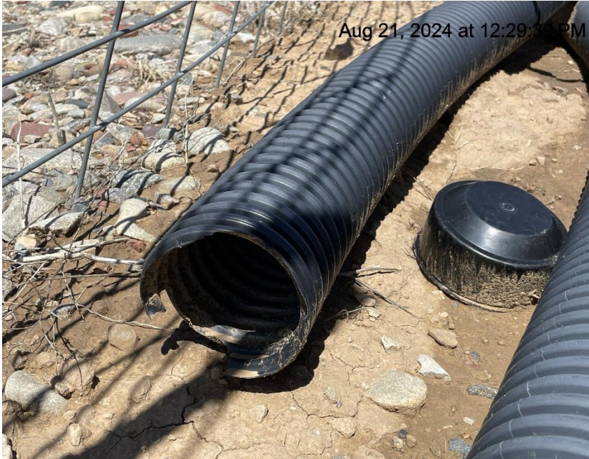
Photo # 5786 Flowline heating insulation open ended /wildlife hazard/available for entry by wildlife
