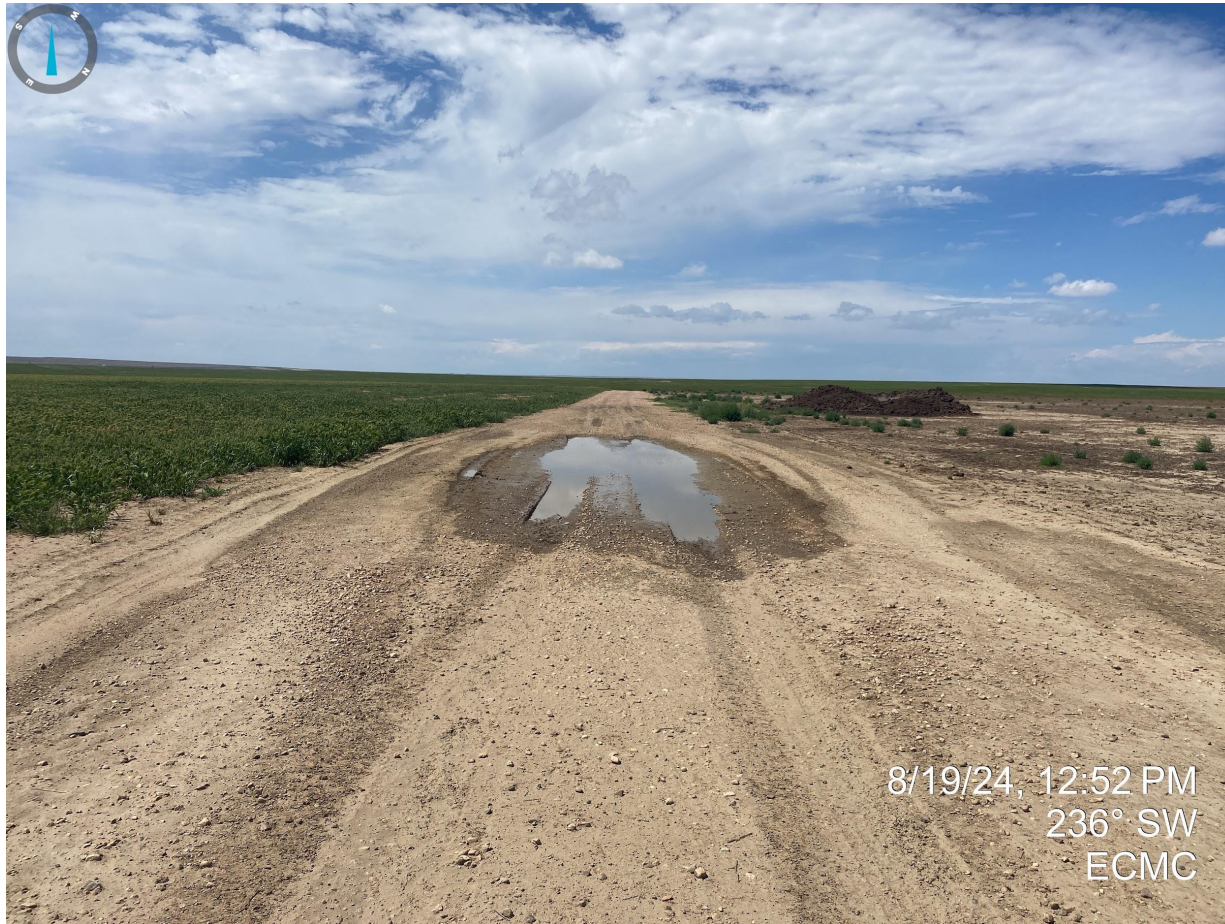
Photo 14. Maintenance advised along access road to manage stormwater and prevent trackout, and to reduce access road expansion.
