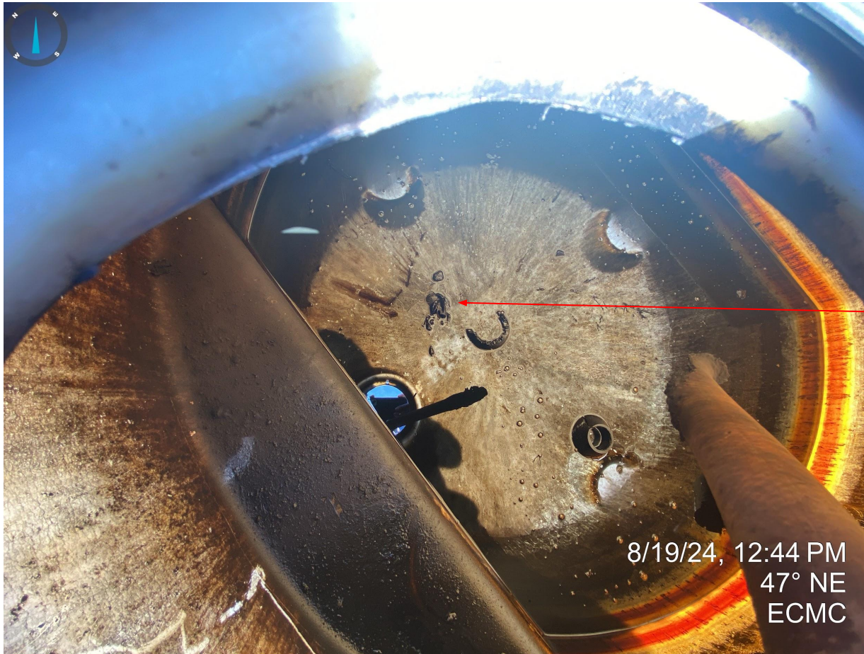
Photo 9. Tank/Container at flare unit does not have adequate wildlife BMPs to prevent or exclude entry by wildlife. Red arrow indicates wildlife mortality (unidentified bird) within container contents. Oily waste shall be removed and wildlife BMPs installed.
