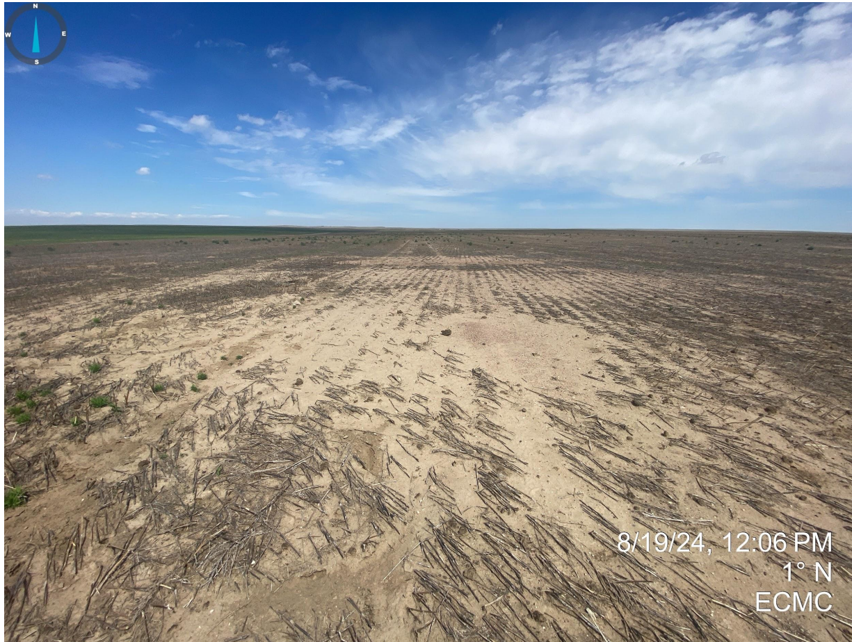
Photo 1. Road Base material remains throughout the location, which does not appear to have been contoured and graded to reflect adjacent topography.
