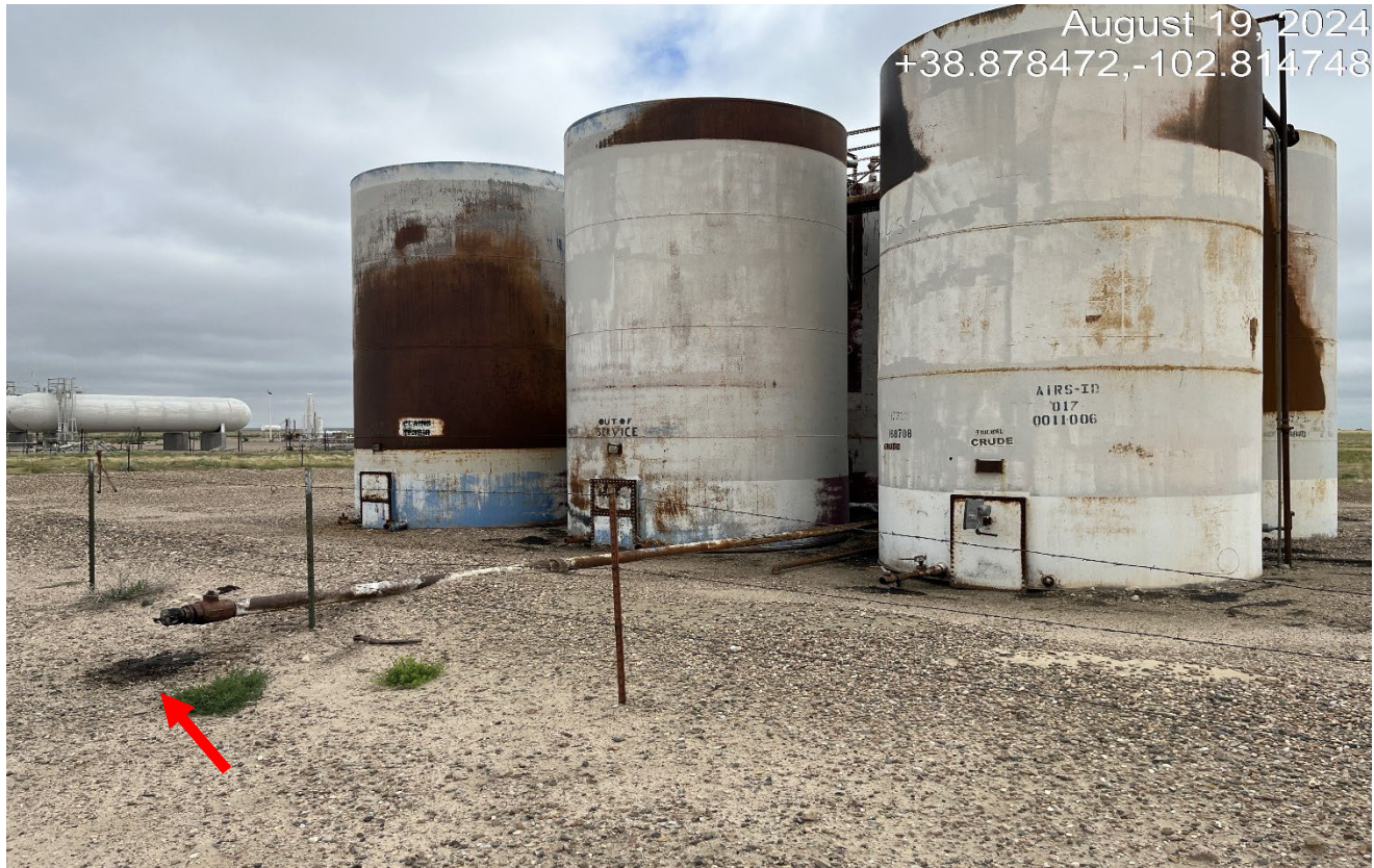
Photo 2. Facing northeast toward the tank battery. The oil stained soils at the outlet have not been cleaned up. Tanks labels are missing or peeling off.
