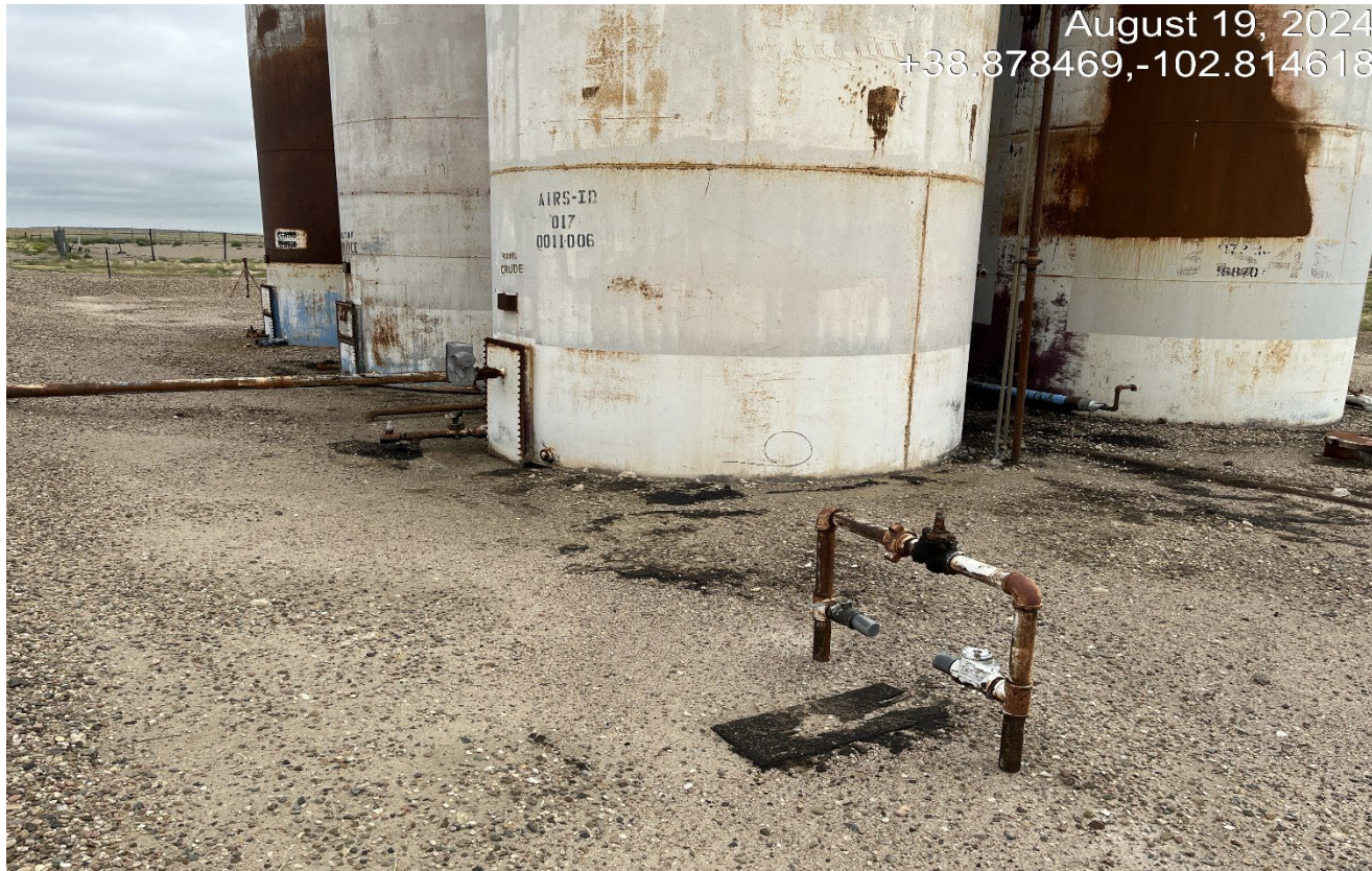
Photo 3. There is oil stained soils between the tanks from a previous spill. This will need to be reported and cleaned up.
