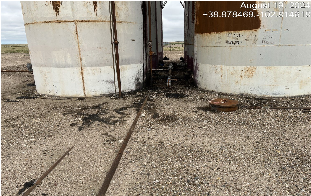
Photo 4. There is oil stained soils between the tanks from a previous spill. This will need to be reported and cleaned up.
