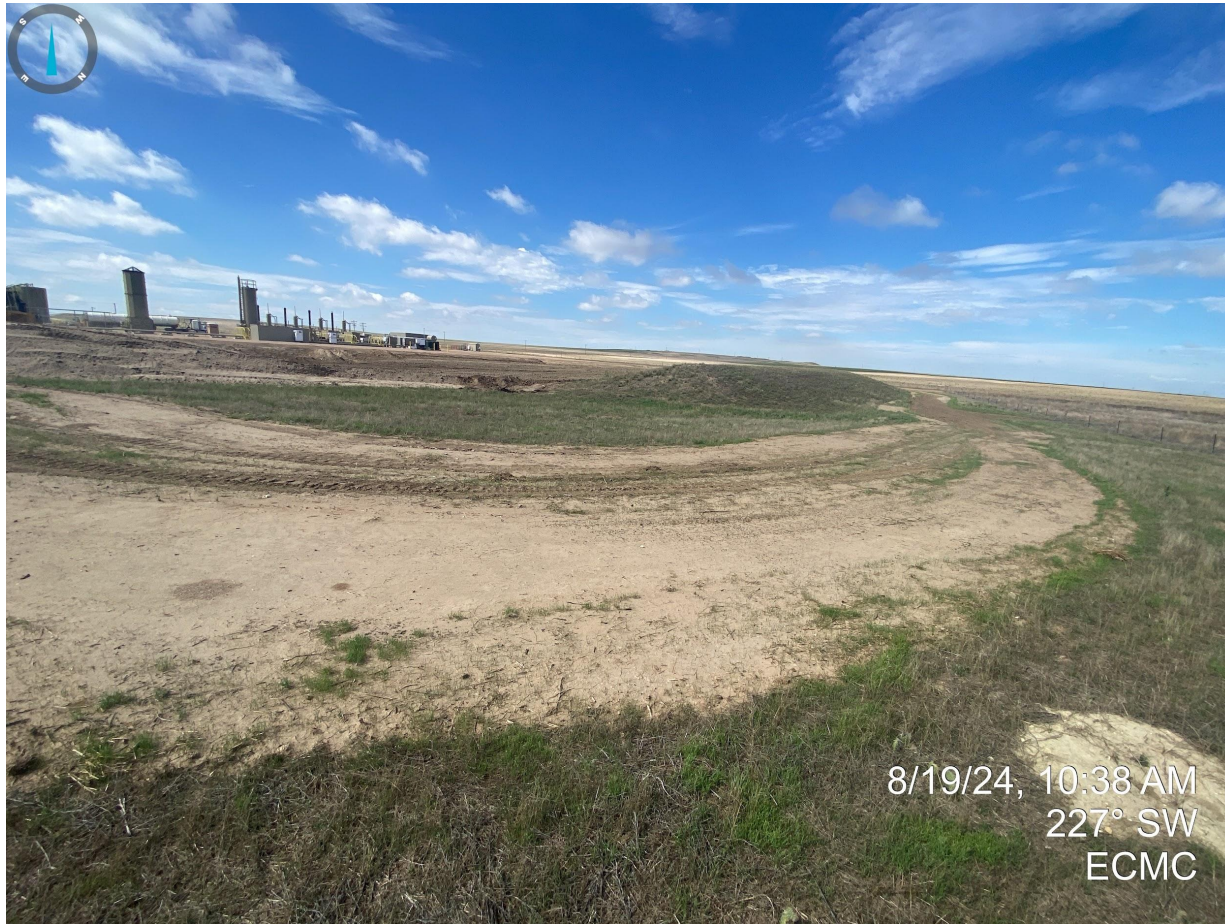
Photo 8. Northeast corner of the disturbance area. Photo illustrates that perimeter stormwater controls (ditch and berm) have been uninstalled/removed at the time of this inspection.
