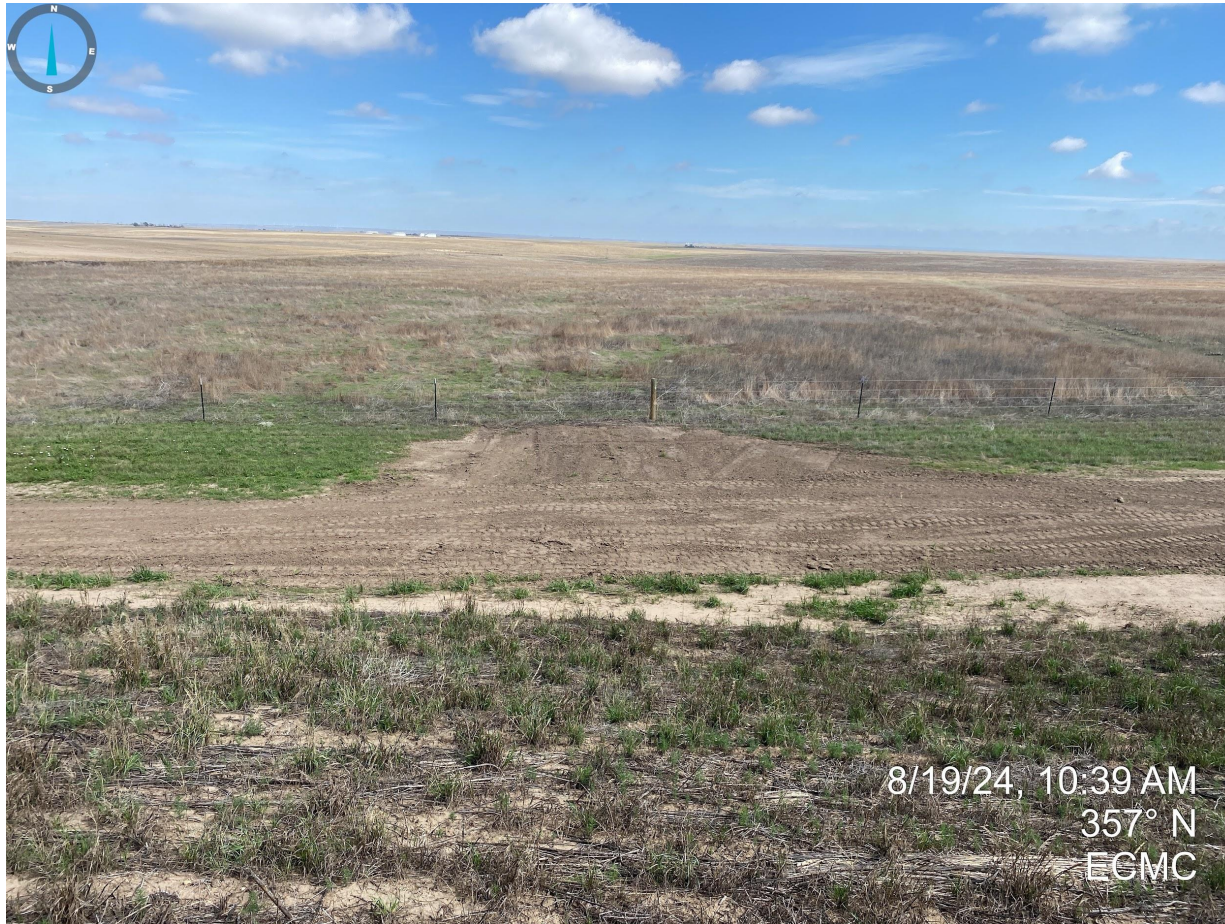
Photo 9. Northern/center portion of the disturbance area. Photo illustrates that stormwater control measures (ditch and berm, sediment trap) have been uninstalled/removed at the time of this inspection.
