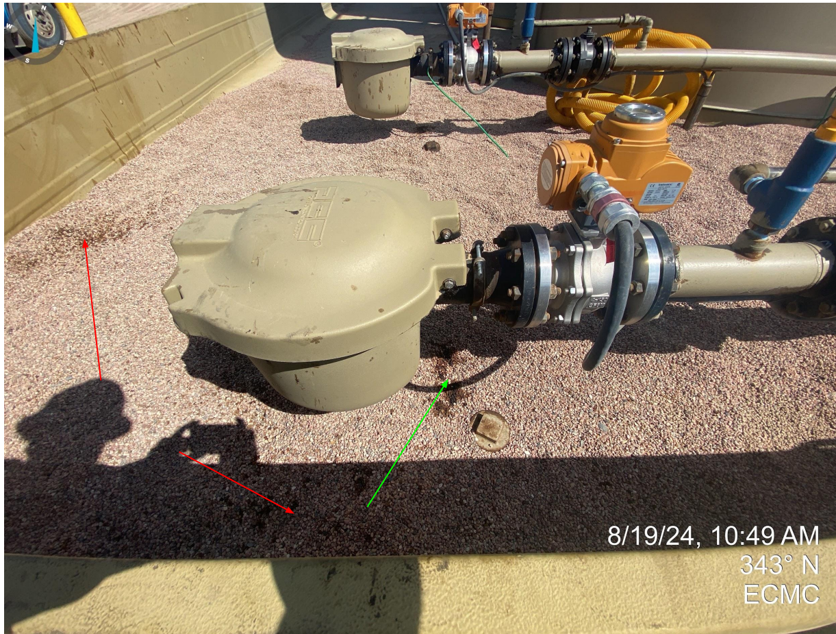
Photo 19. Green arrow indicates previous discovery of stained soil observed on FIR doc# 708201482 (Photo 5 of inspection photos) which does not appear to have been removed. Red arrows indicate stained soil observed at time of this inspection.
