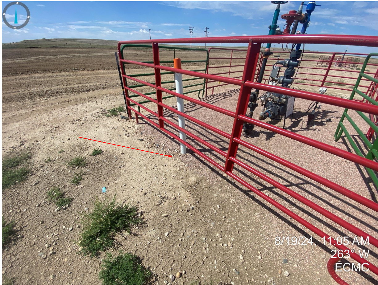
Photo 24. Previous subsidence at Well API 123-50755 appears to have been backfilled and repaired.
