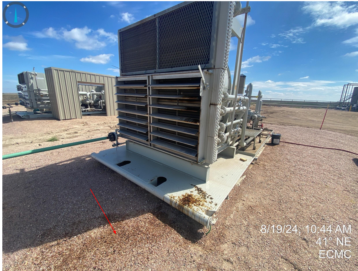
Photo 15. Stained soil observed at compressor station; leak appears to be coming from compressor fan/coils.
