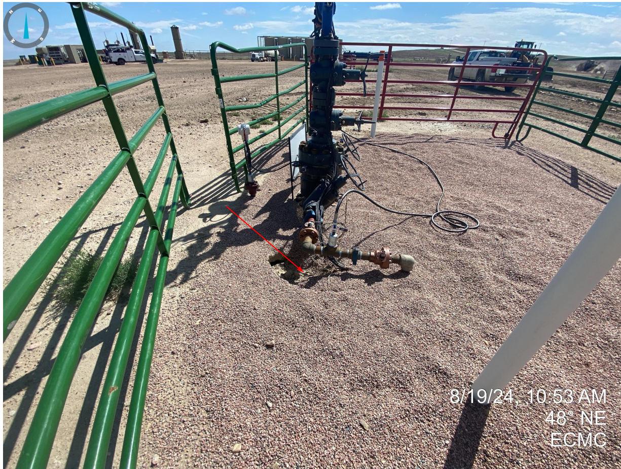
Photo 23. Subsidence observed at Well API 123-50750.
