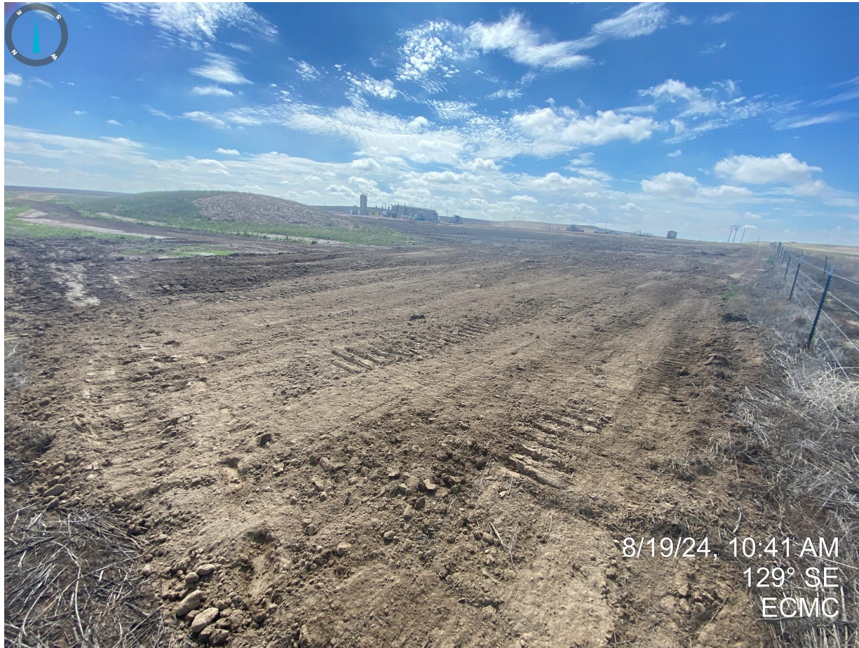
Photo 11. Taken from the northwest corner of the disturbance area. Photo illustrates that the sediment trap has been uninstalled/removed.
