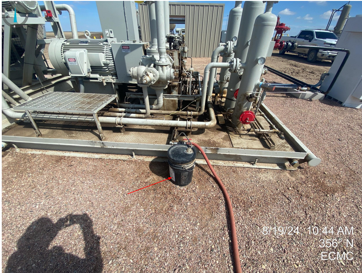
Photo 16. 5 gallon bucket outside of secondary containment.
