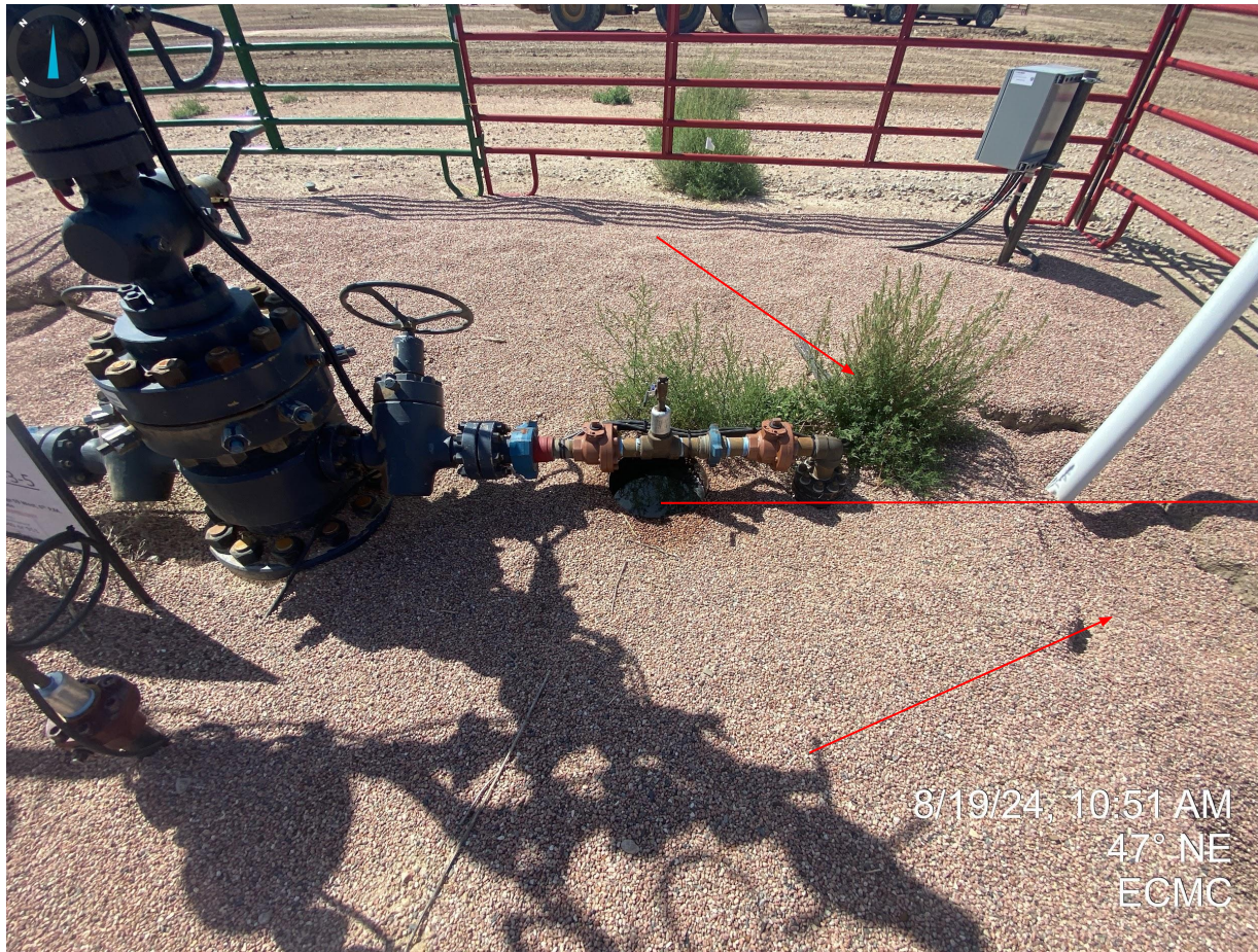
Photo 21. Continued from Photo 20. Undesirable vegetation, subsidence and unidentified fluid within mouse/rat hole.
