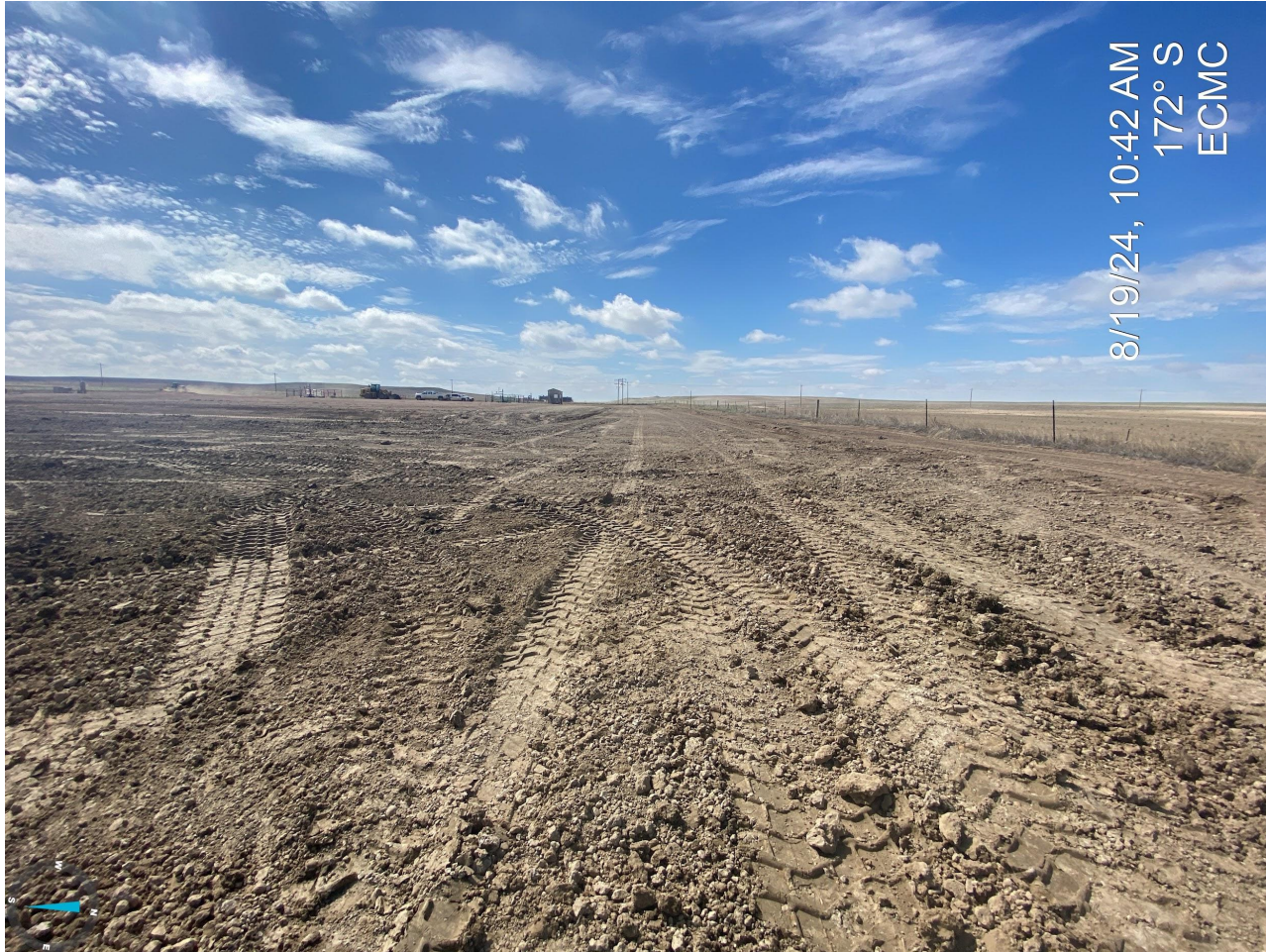
Photo 14. Taken from the western portion of the disturbance area. Photo illustrates that stormwater controls measures (perimeter ditch and berm, and sediment traps) have been removed/uninstalled.
