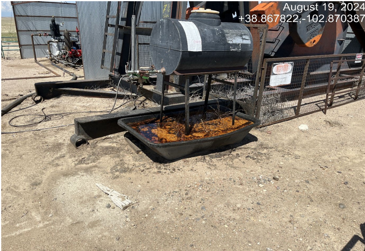
Photo 2. The secondary containment is filly of oily fluid and needs to be drained and removed. Netting needs to be installed to prevent wildlife entry.
