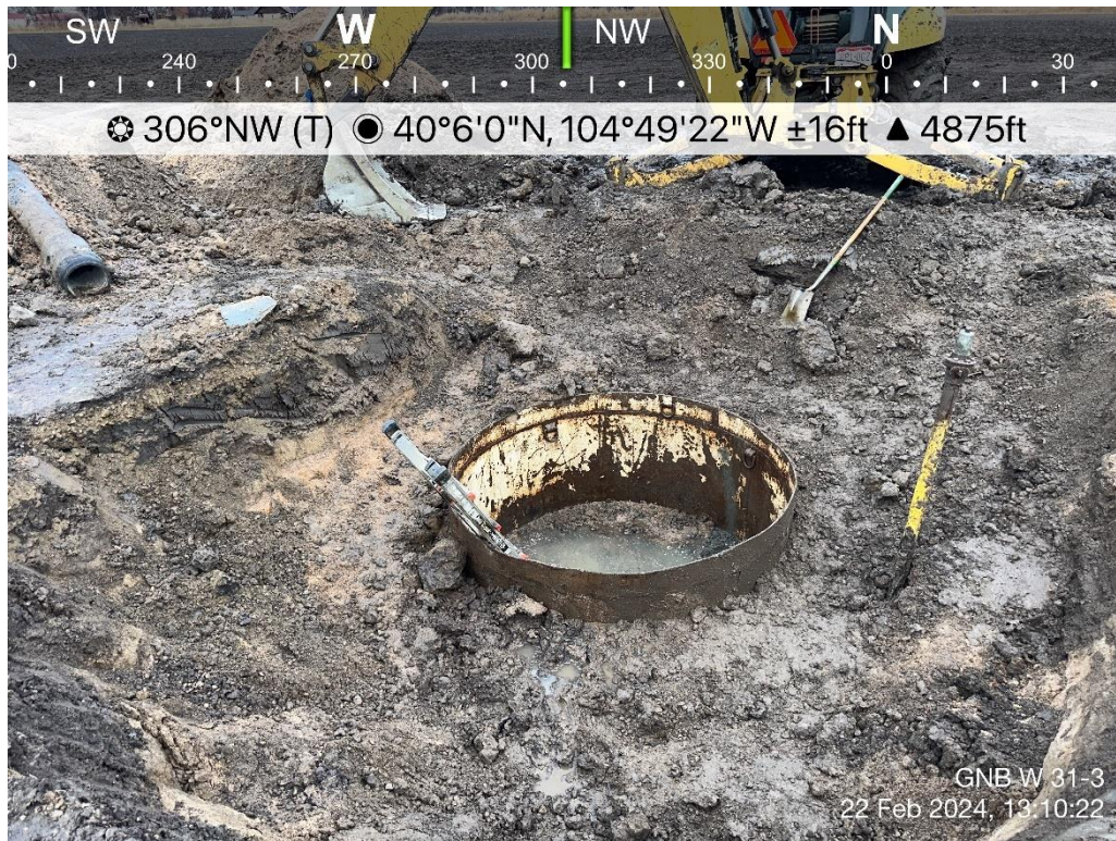
Wellhead Excavation (Groundwater Present)
