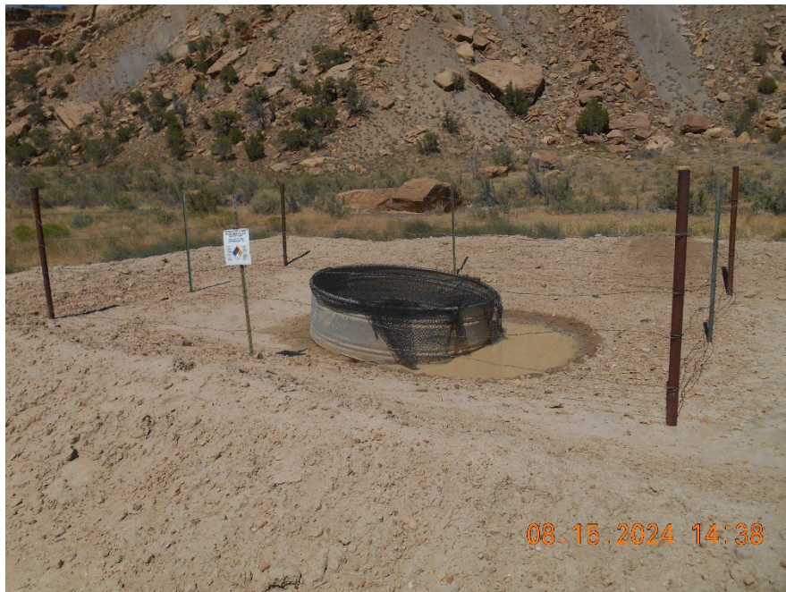
Blowdown tank with fence
