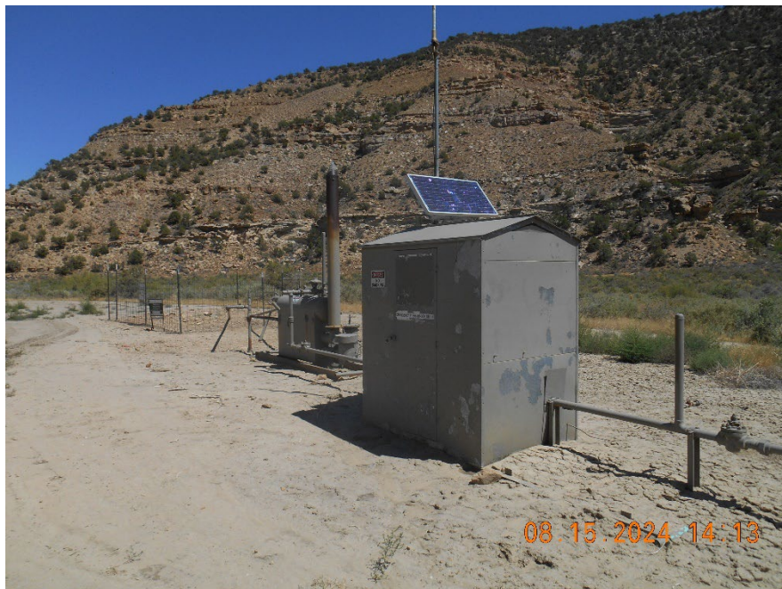
Separator and Meter housing
