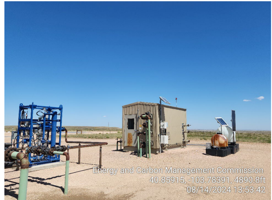
Photo 14 – Gas Lift Injection Meter House
