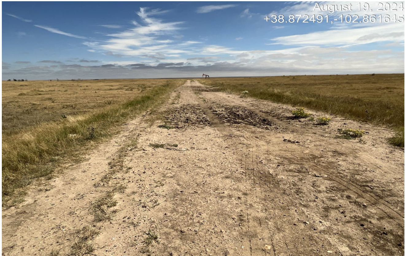
Photo 1. There is road damage which vehicle are avoid which is widening the road. This must be repaired and stabilized.
