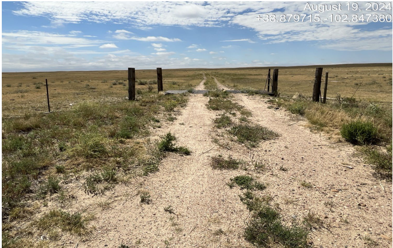
Photo 1. Facing south at the beginning of the access road. The cattleguard will need to be removed and fence installed back to original position. The road needs to be reclaimed.
