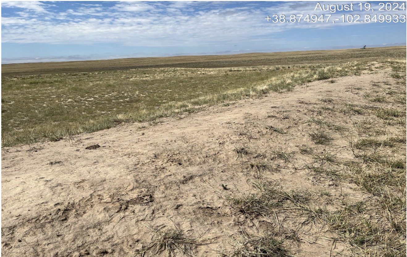
Photo 6. Facing southwest at the top of the cut slope. There is a berm along the top of the which needs to be recontoured along the cut slope
