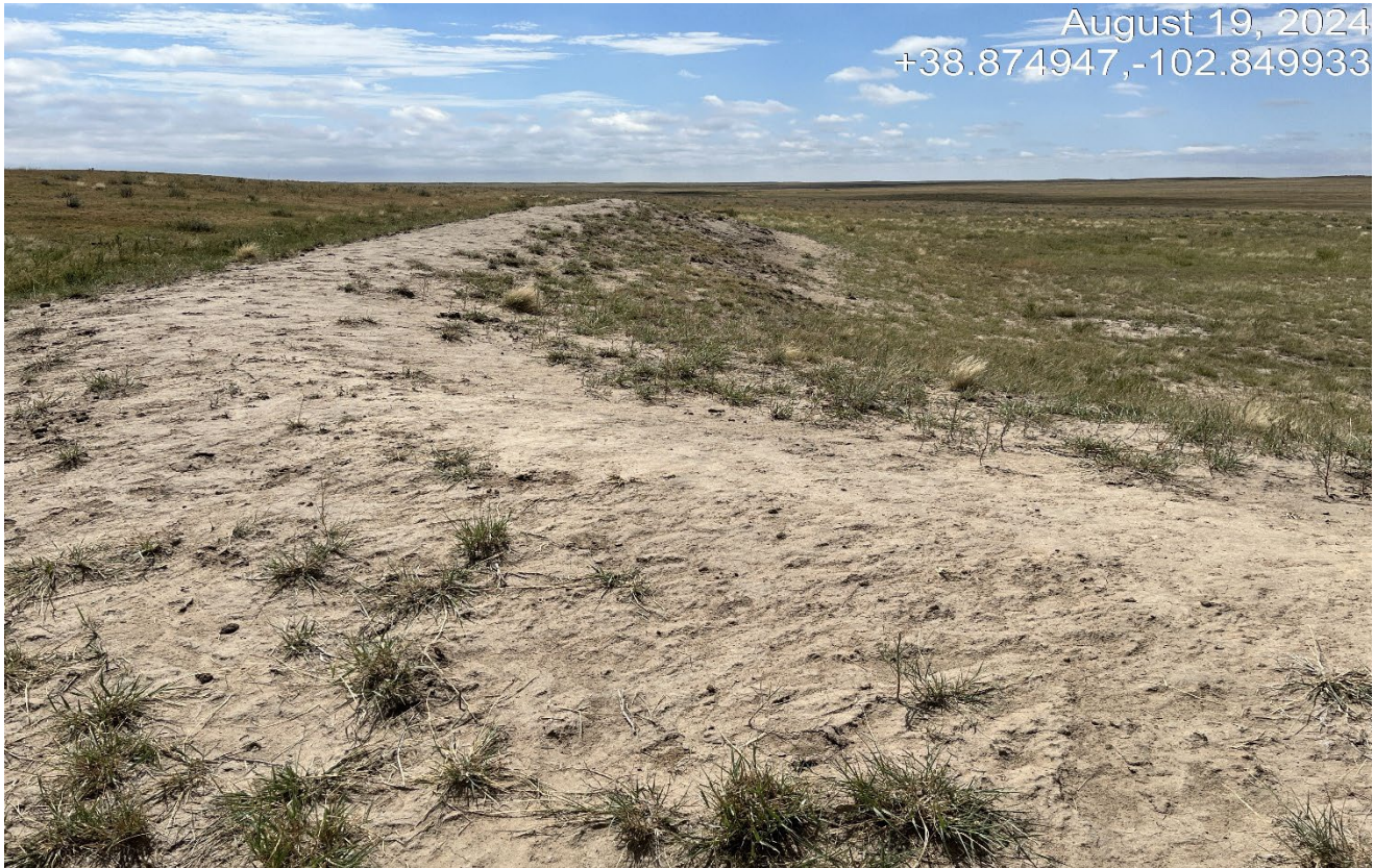
Photo 5. Facing south at the top of the cut slope. There is a berm along the top of the which needs to be recontoured along the cut slope
