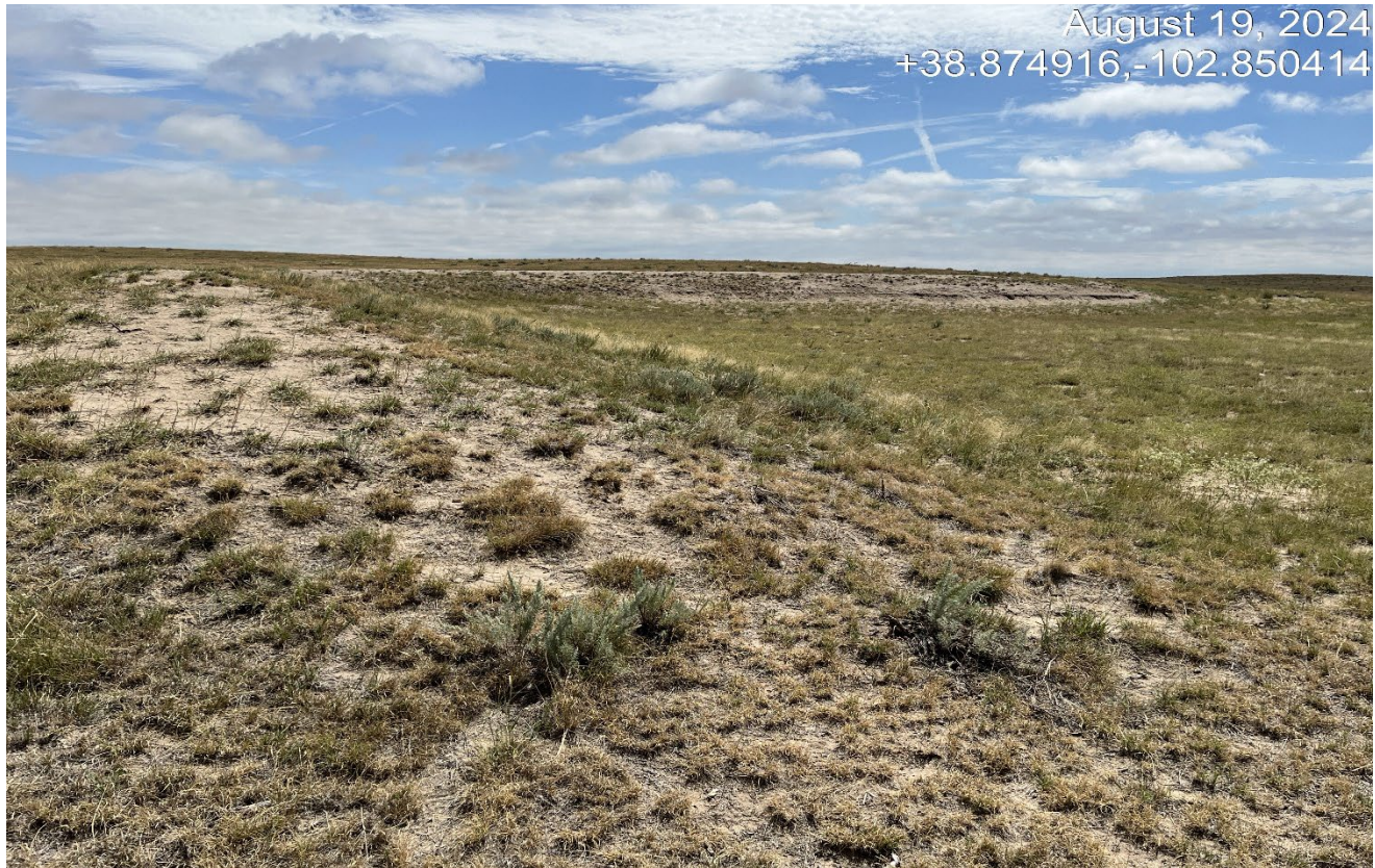
Photo 7. Facing southeast at the top of the cut slope. There is a berm along the top which needs to be recontoured along the cut slope.
