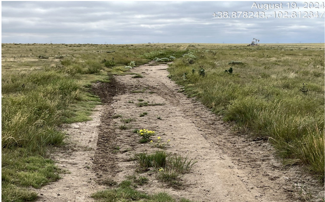
Photo 2. Facing southeast along the access road. Vehicles are causing unnecessary disturbance driving outside of the access road due to stormwater pooling on the road. The access road must be maintained and vehicles shall not drive outside of the access road
