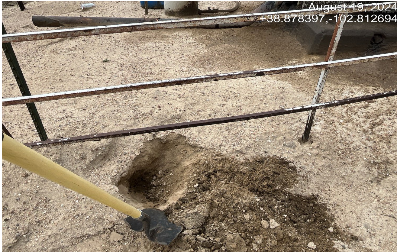
Photo 7. It appears there was sand spread on top of the spill which was not cleaned up per the rules. There is still oily soils that remain underneath the sand that was placed over the stained soils.
