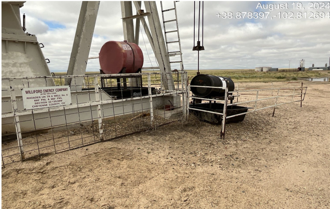
Photo 9. There is oily fluid in the secondary containment and no wildlife protection/netting is installed. The labeling on the barrels is faded and needs to be updated.
