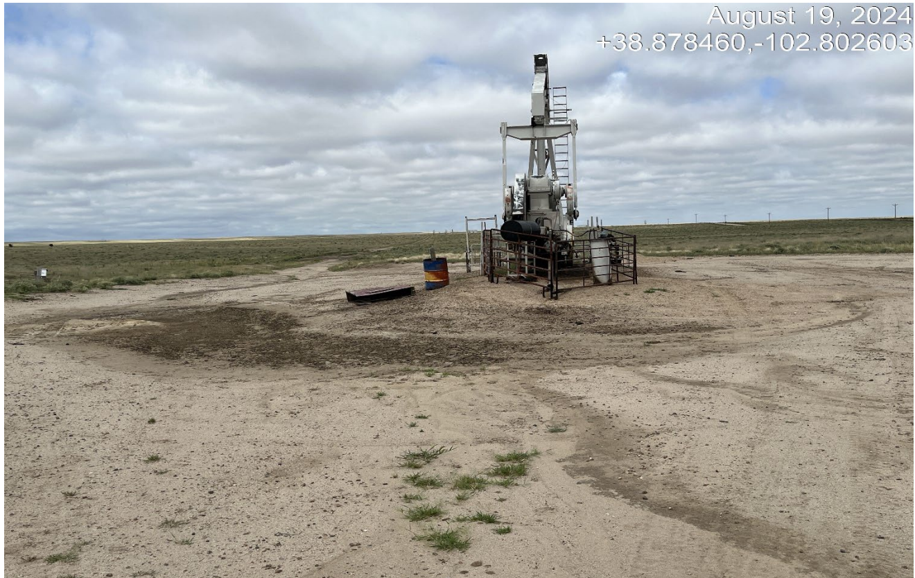
Photo 7. Facing west toward the location. There is evidence of water pooling at the east side of the pumpjack with no proper drainage. There is a piece of the pumpjack laying on the ground.
