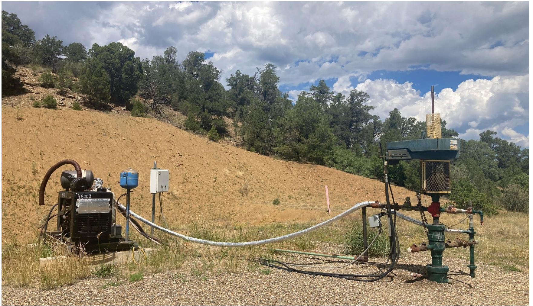
PHOTO 3: WELLHEAD AND EQUIPMENT
