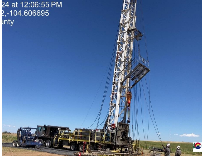
Pic 1 Rig crew rigging up rig
