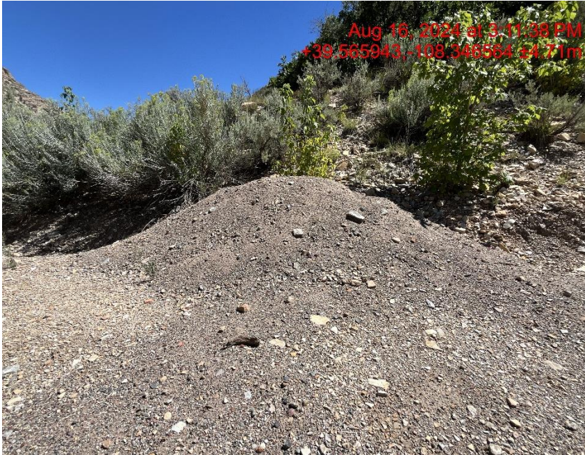
Stockpiled soils with no BMP's - Photo #04821
