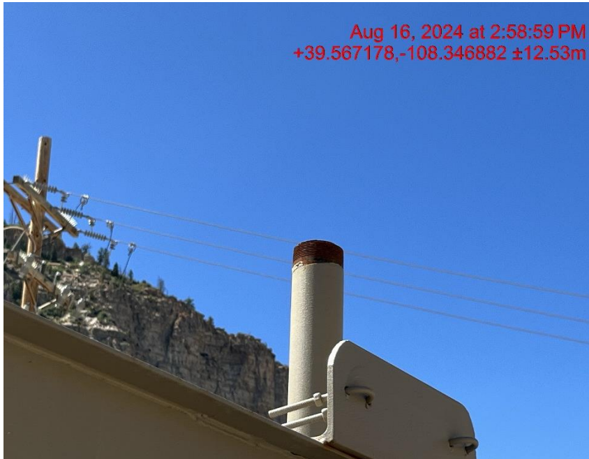
PRV line not capped - Photo #04803
