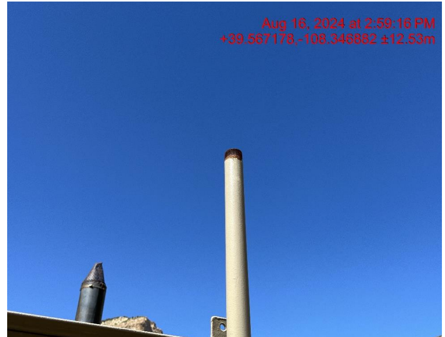
PRV line not capped - Photo #04804
