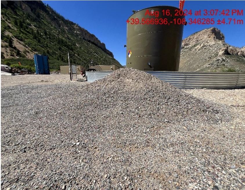
Stockpiled soils with no BMP's - Photo #04812
