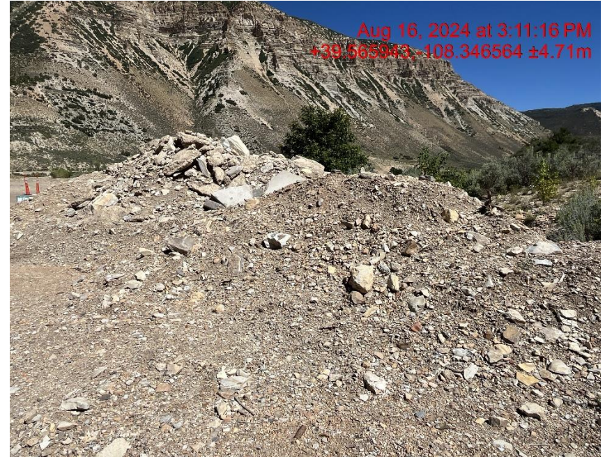
Stockpiled soils with no BMP's - Photo #04818
