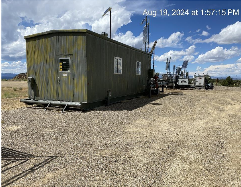
Production pad looking Northwest
