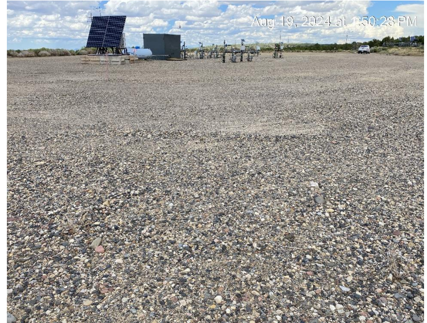
Well pad from Southwest corner
