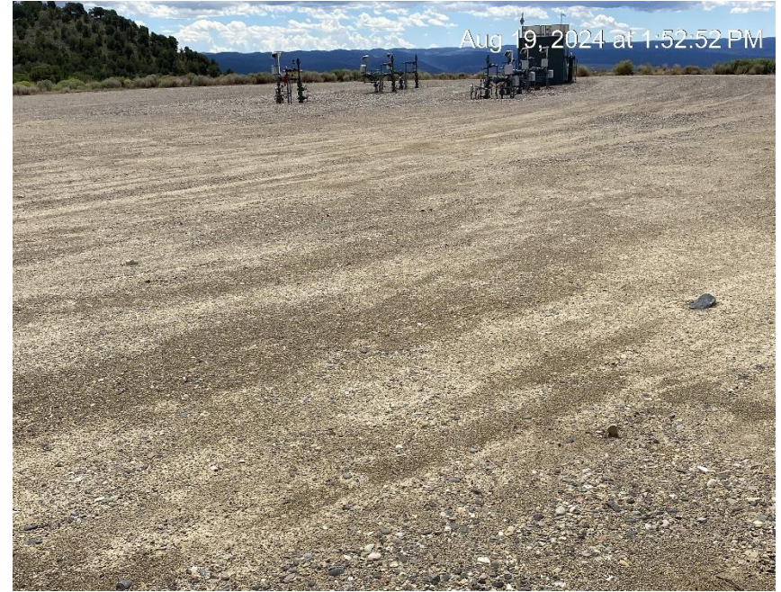
Well pad from Northeast corner
