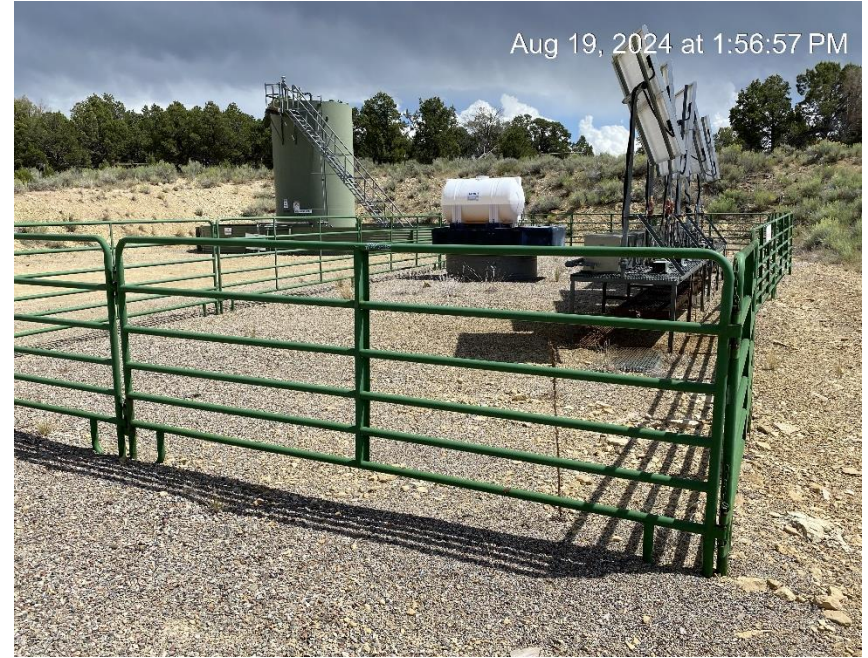
Production pad looking Southeast
