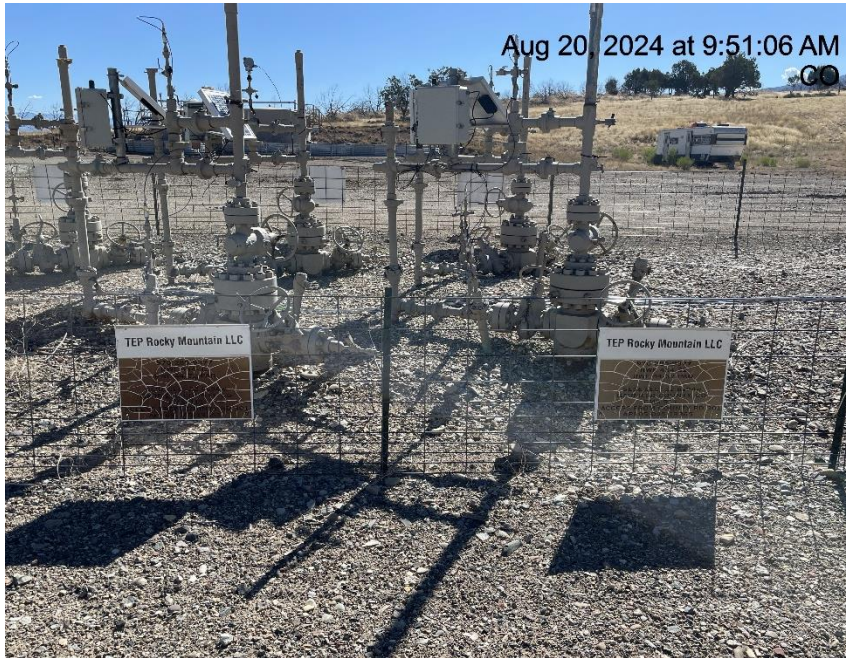
Photo # 5483 Wellhead signs weathered & cracking/starting to become illegible
