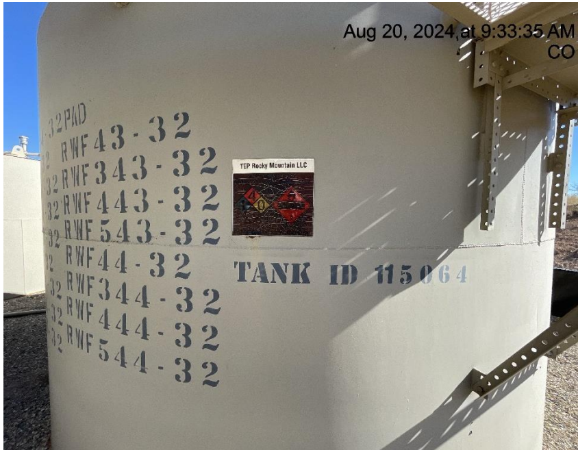
Photo # 5481 Tank label weathered & some required info is illegible
