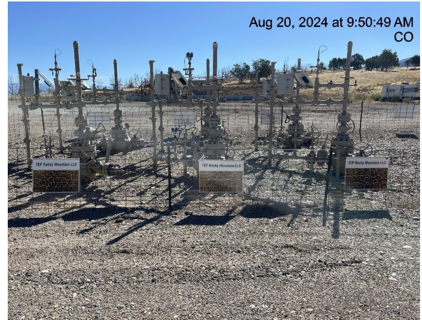
Photo # 5482 Wellhead signs weathered & cracking/starting to become illegible
