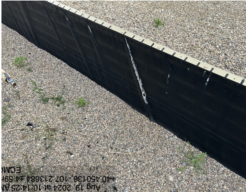
Holes in secondary liner
