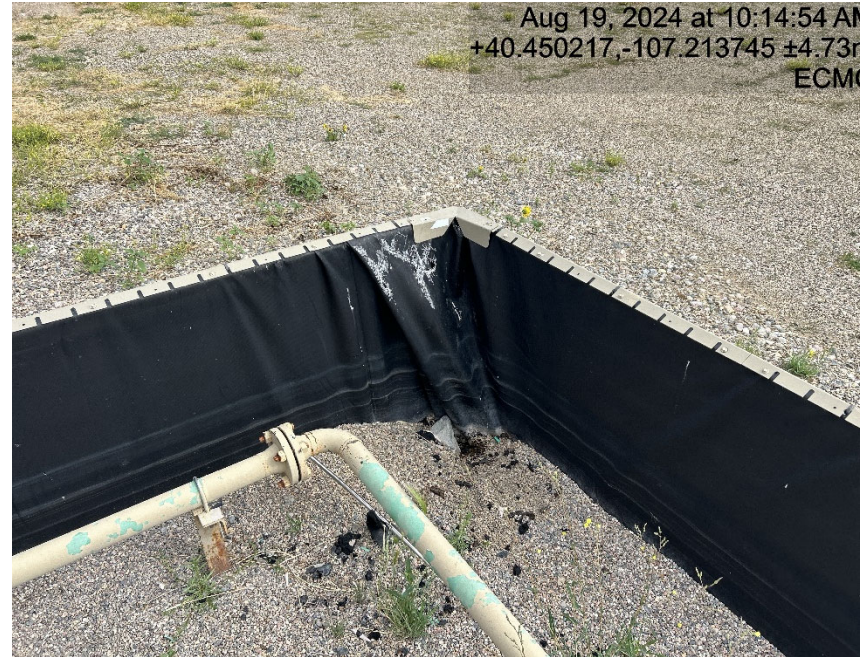
Holes in secondary liner
