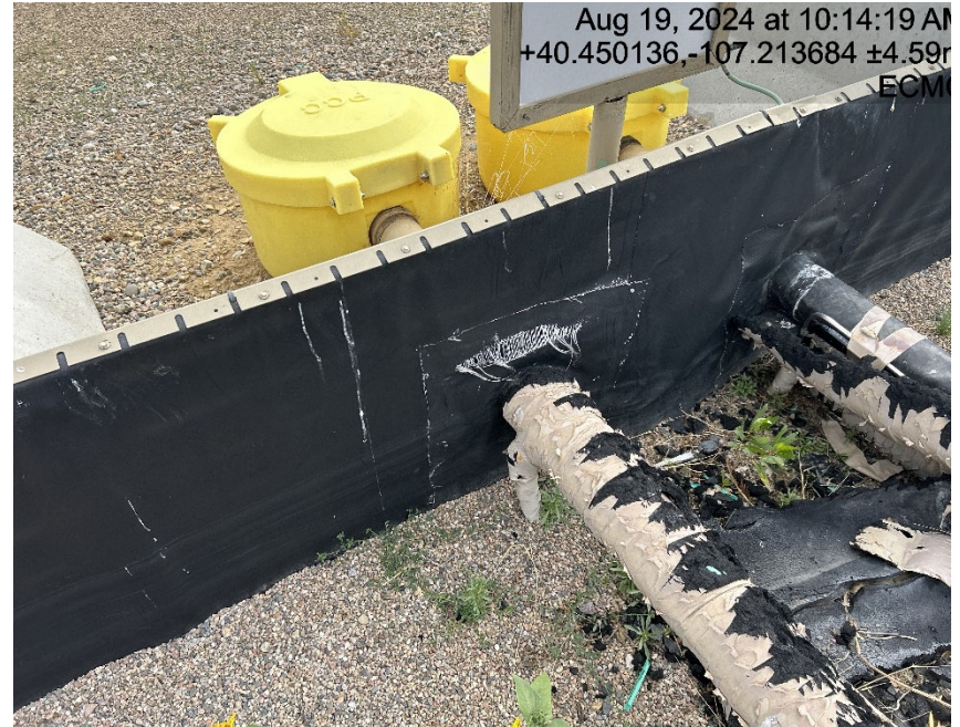
Holes in secondary liner
