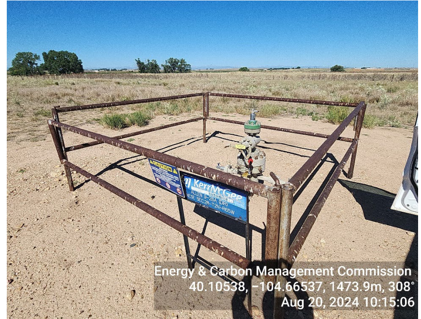
Photo 6: TA Wellhead
