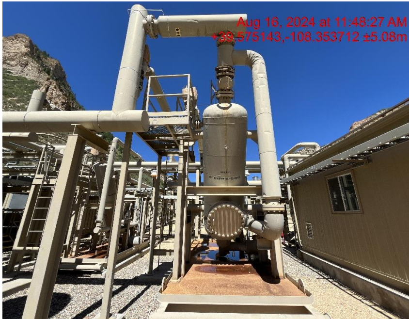
Sand Separator/out of service - Photo #04701
