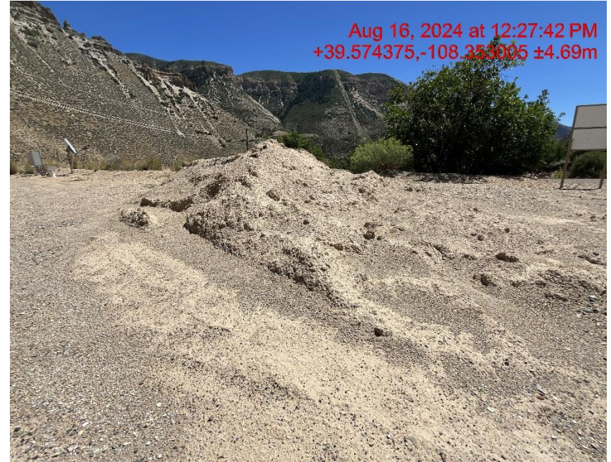
Stockpiled soils with no BMP's - Photo #04746
