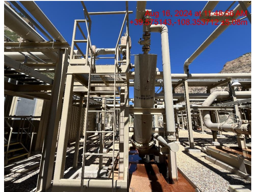
Sand Separator/out of service - Photo #04703
