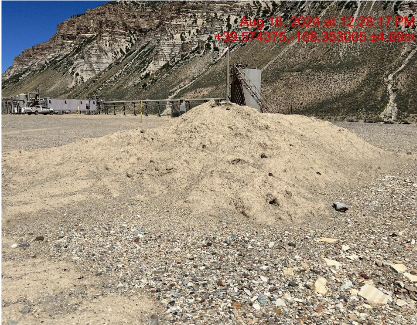
Stockpiled soils with no BMP's - Photo #04747
