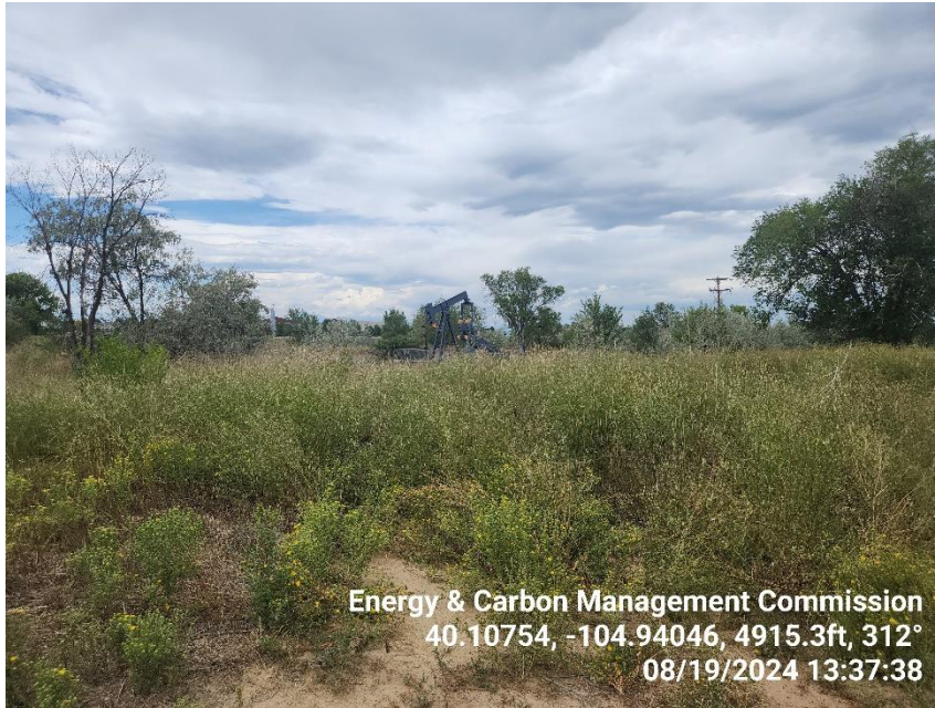
Photo 1 Location access road overgrow with vegetation
