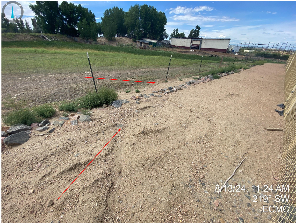
Photo 15. Erosion degradation (riling) along the southern portion of the location, near production equipment.
