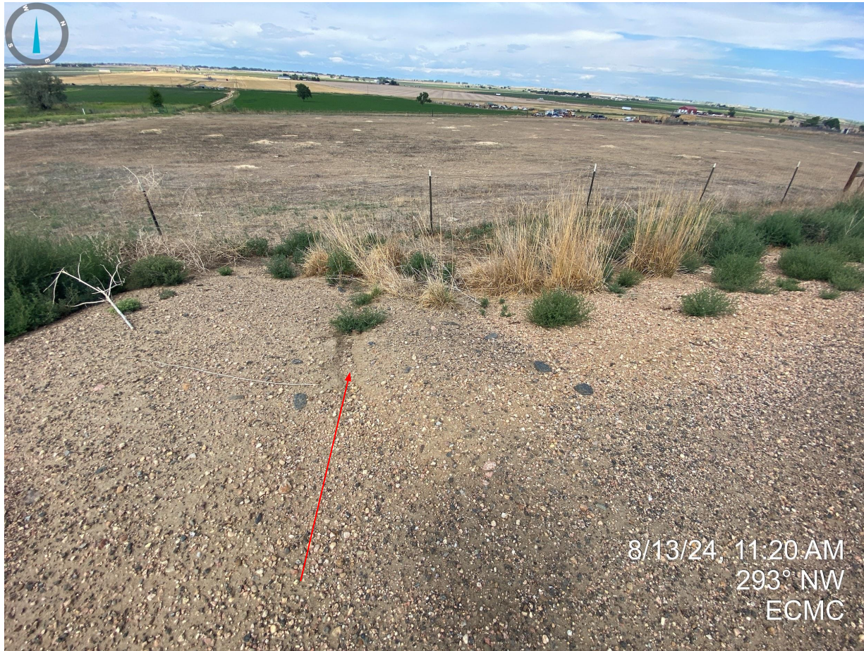
Photo 6. Erosion degradation (riling) observed on the northwest portion of the tank battery.
