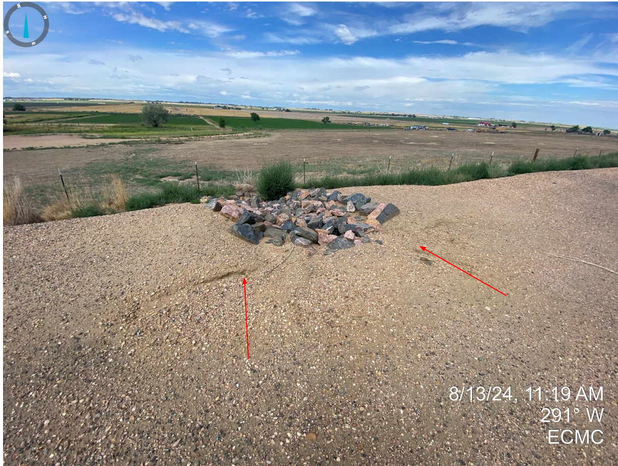
Photo 2. Erosion degradation (riling) observed on the northwest portion of the tank battery.
