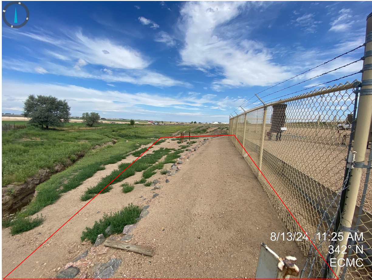
Photo 17. No apparent stormwater control measures observed on the southwest corner of the location, near adjacent irrigation ditch.
