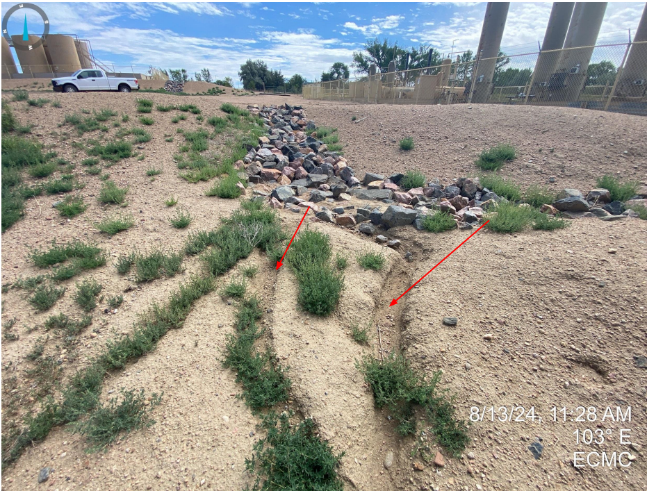
Photos 19 & 20. Erosion degradation and evidence of off location sediment transport observed on the northwest portion of the fenced production equipment.
