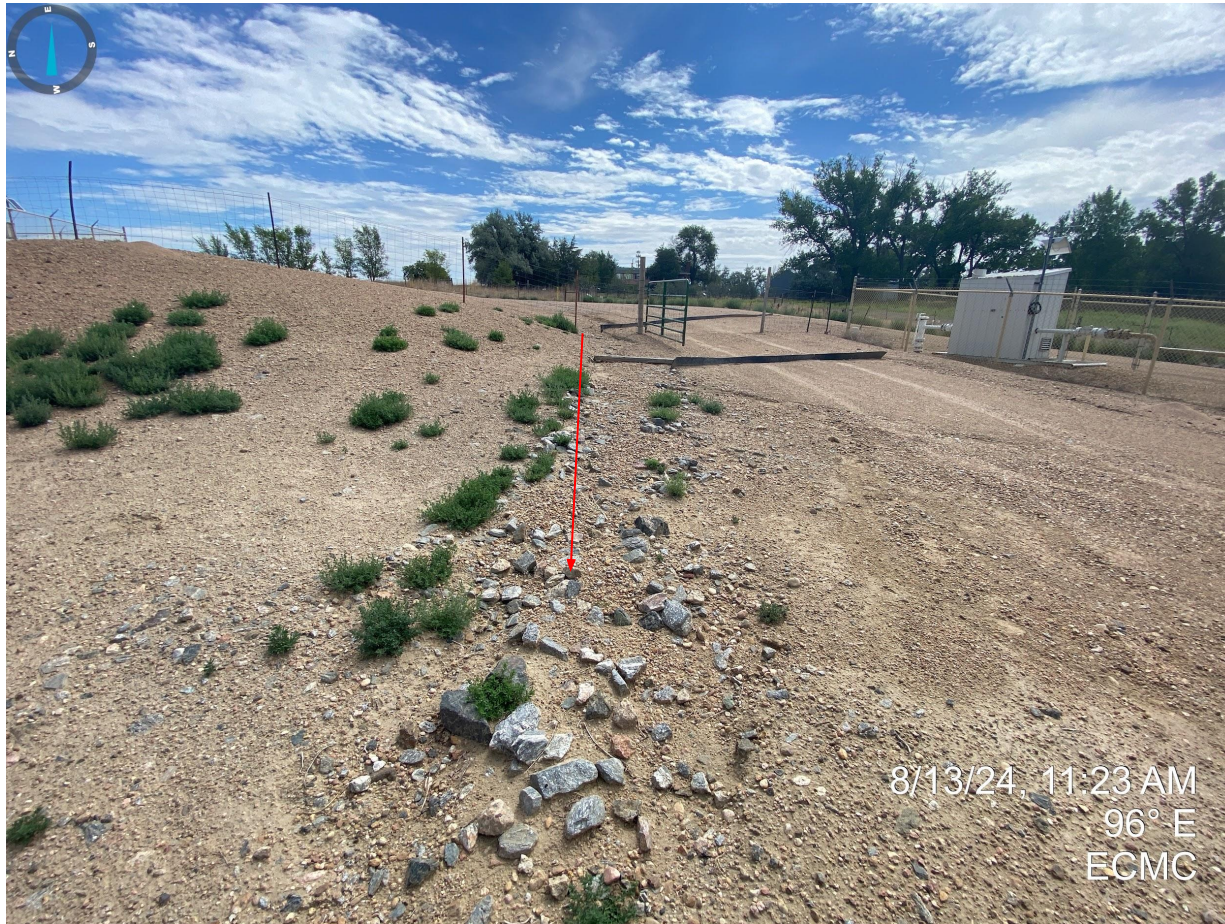
Photo 13. Continued from Photo 12; photo illustrates sediment transport onto lower portions of the access road/production areas.
