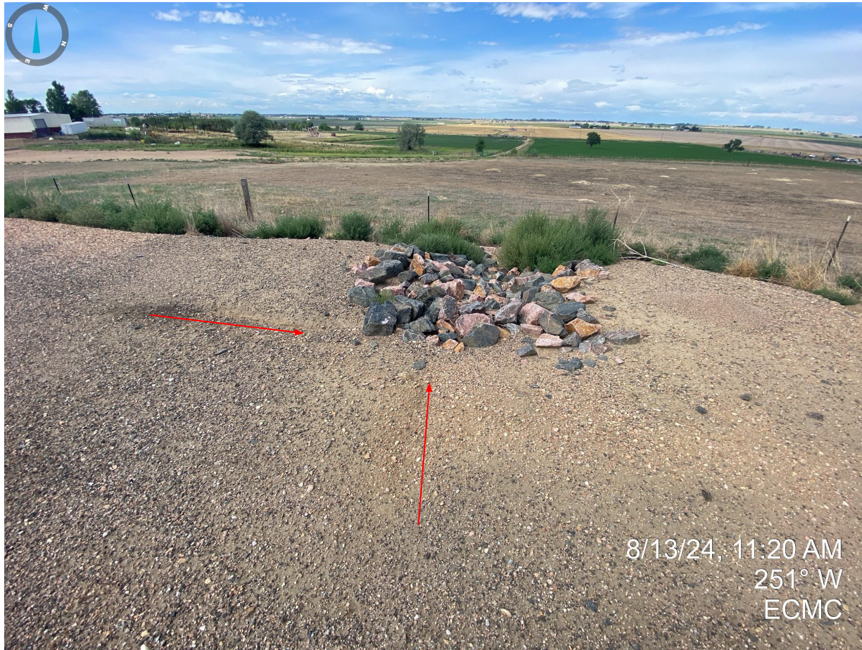
Photo 5. Erosion degradation (riling) observed on the northwest portion of the tank battery.
