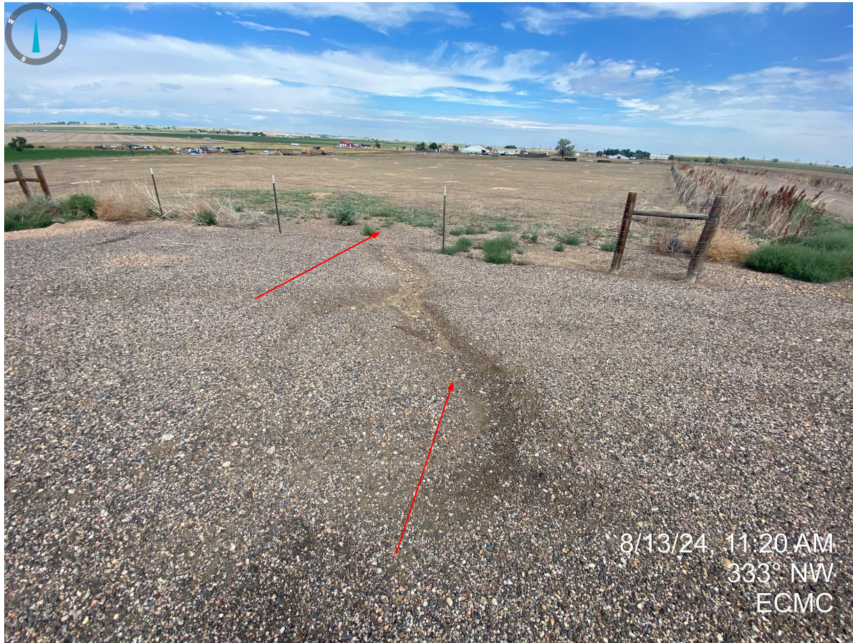
Photo 7. Erosion degradation (riling) and sediment transport into adjacent lands observed on the north portion of the tank battery.
