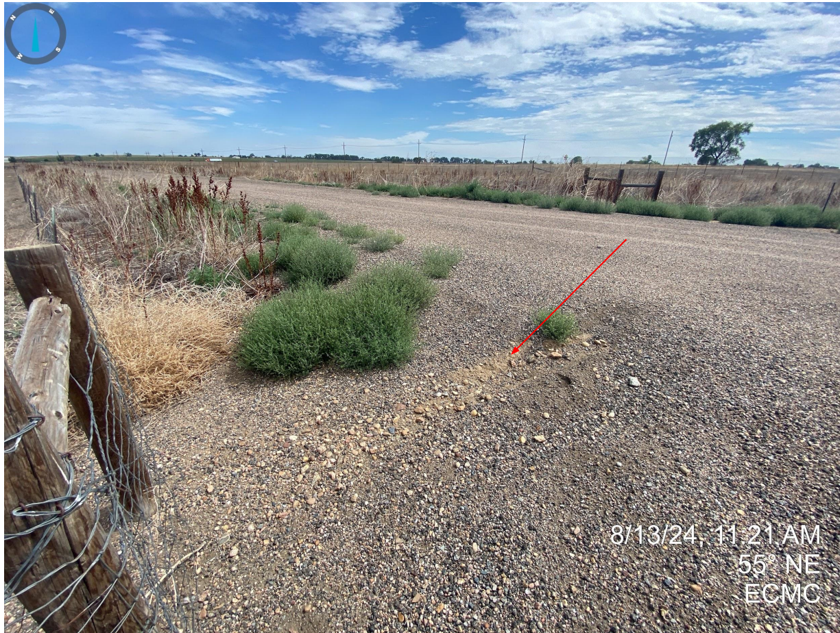
Photo 9. Erosion degradation and undesirable vegetation along the location's access road.
