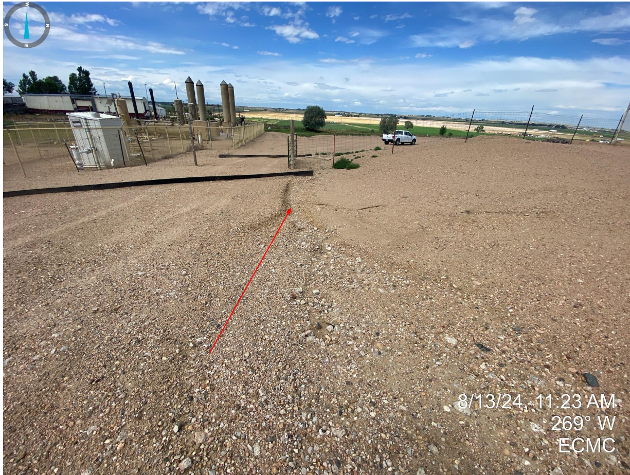
Photo 12. Erosion degradation observed south of the tank battery.
