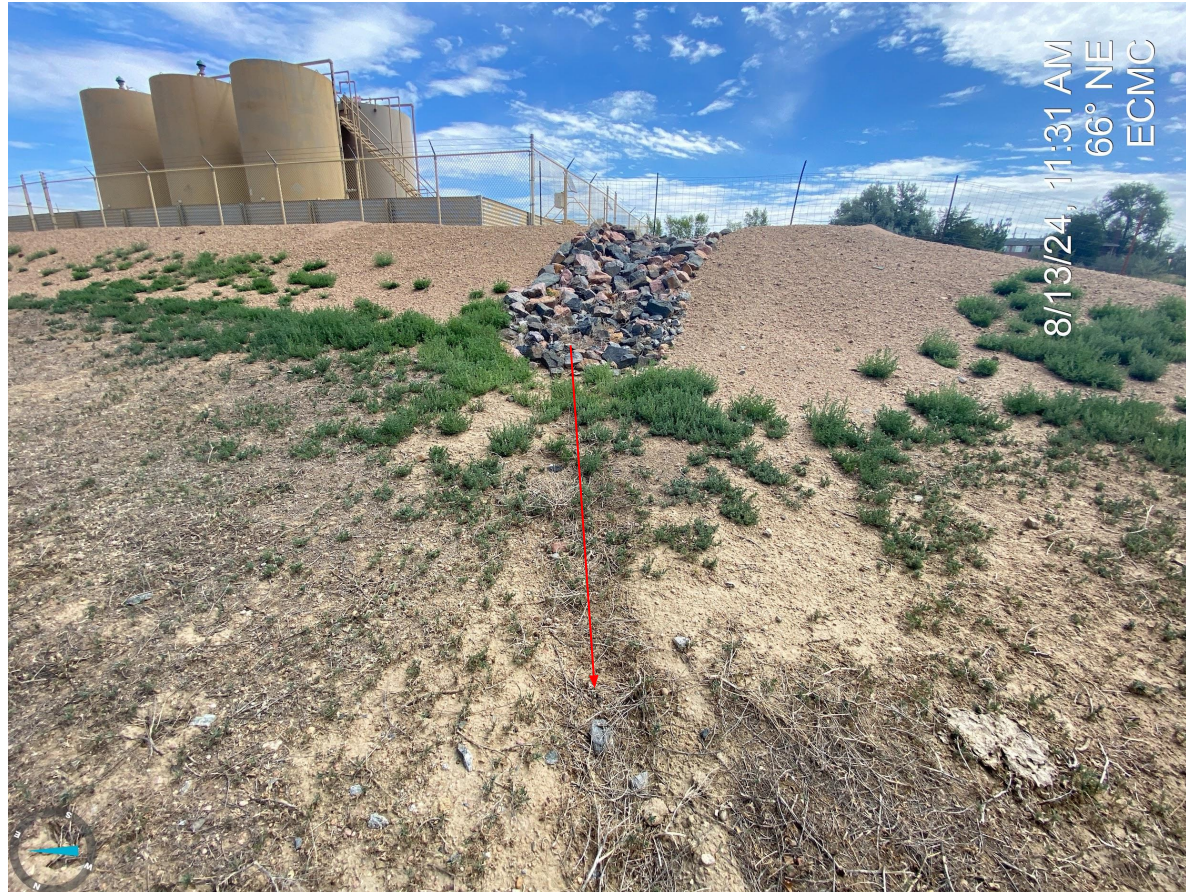
Photo 23. Erosion degradation observed at the outlet of control measure.
