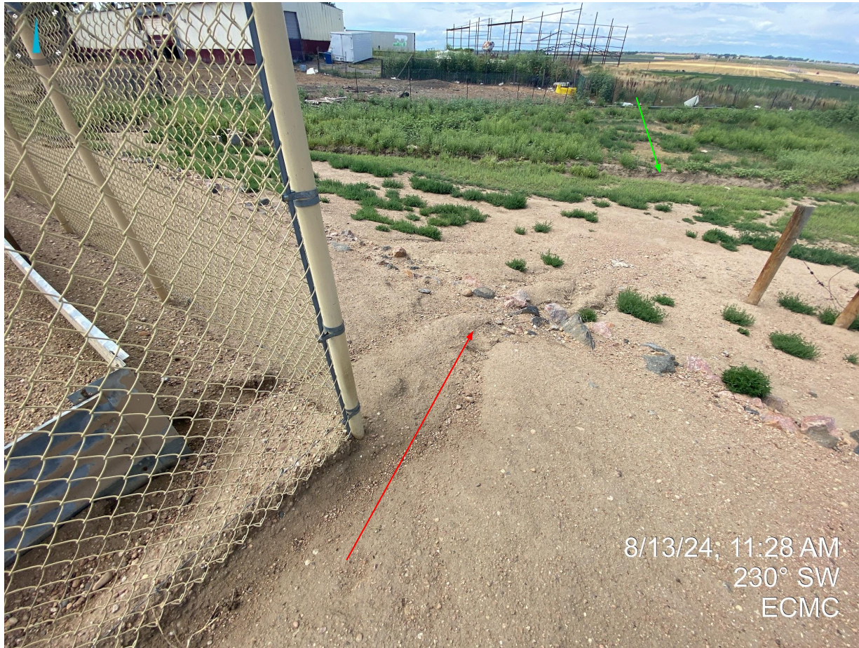
Photo 18. Erosion degradation observed on the northwest corner of fenced production equipment; no apparent stormwater control measures near adjacent irrigation ditch (green arrow).
