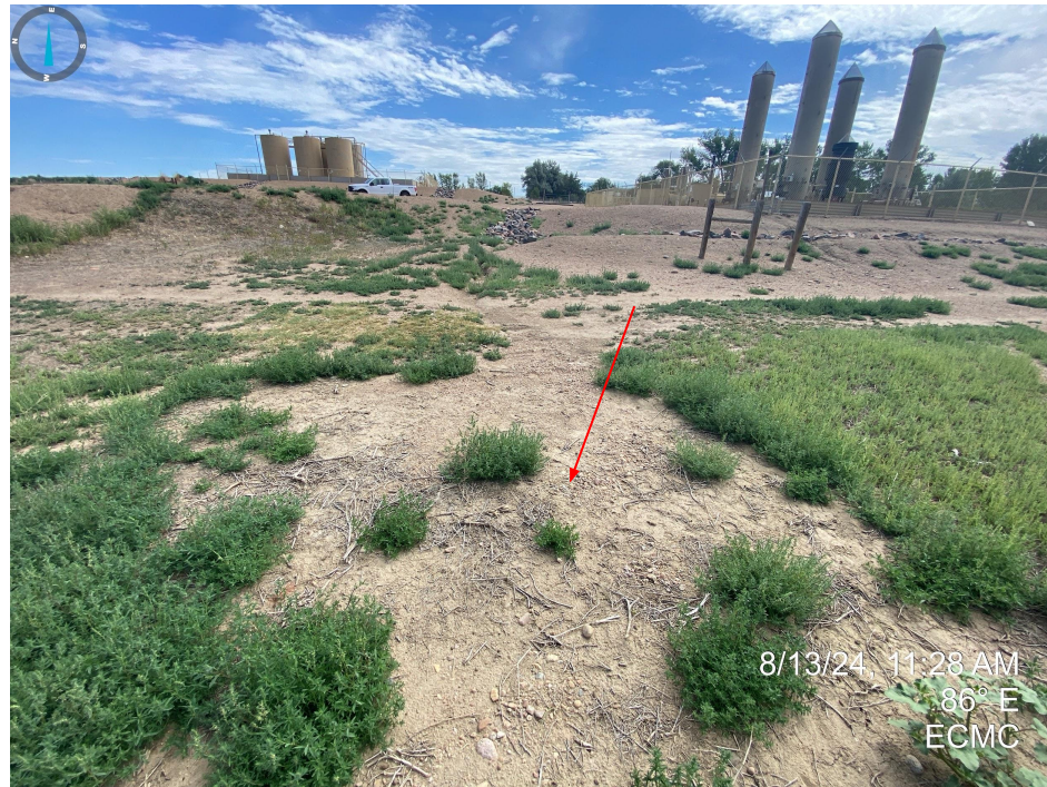
Photos 19 & 20. Erosion degradation and evidence of off location sediment transport observed on the northwest portion of the fenced production equipment.
