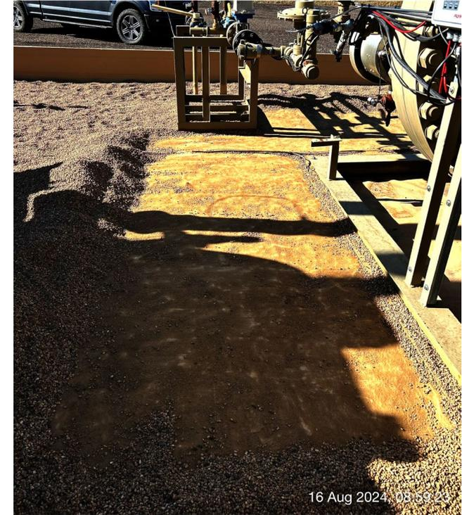
An inspection was conducted on 8/16/2024 and the integrity of the liner was confirmed to be in satisfactory condition. No holes or tears were observed.
