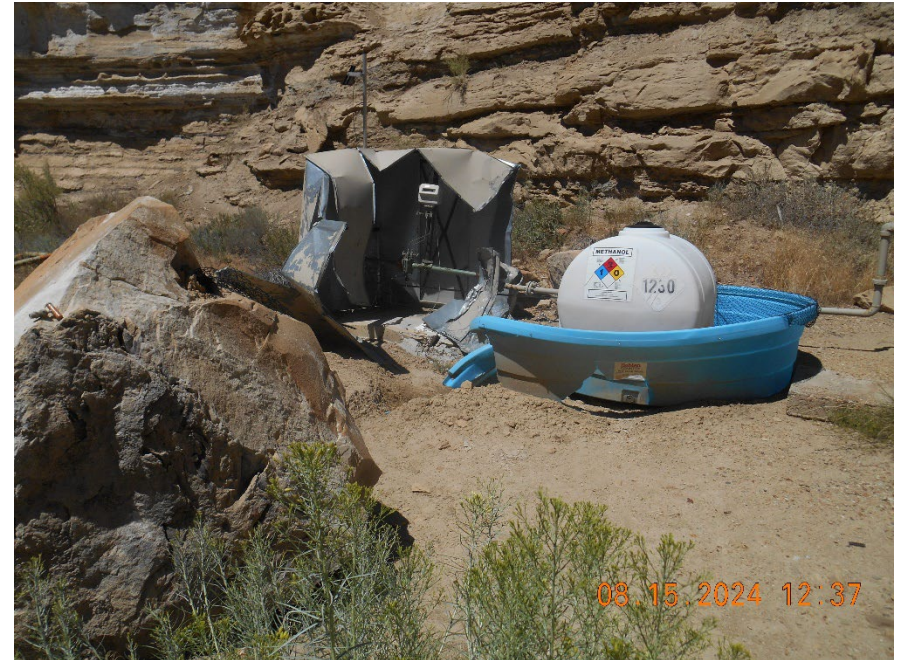
Meter housing and methanol containment destroyed by rock fall
